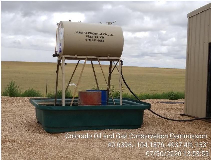
Photo 3 – Day Tank at Compressor missing Wildlife Netting
