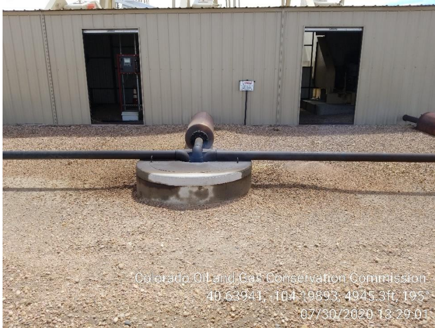
Photo 7 – Stained Soil at Pumping Unit Exhaust
