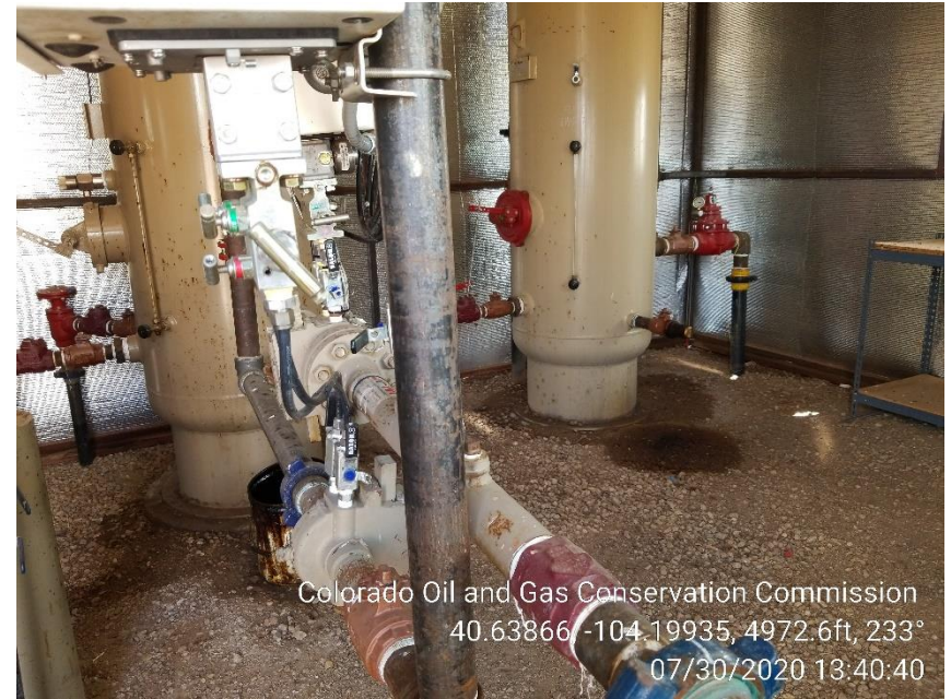
Photo 6 – Stained Soil inside West Heater Treater
