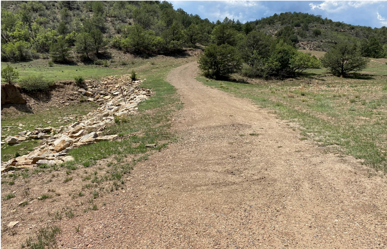
Photo 2. Facing west along the road which passes the drainage. There is concern with the small size of the culverts installed at this drainage crossing however, this area appears to be stabilized.
