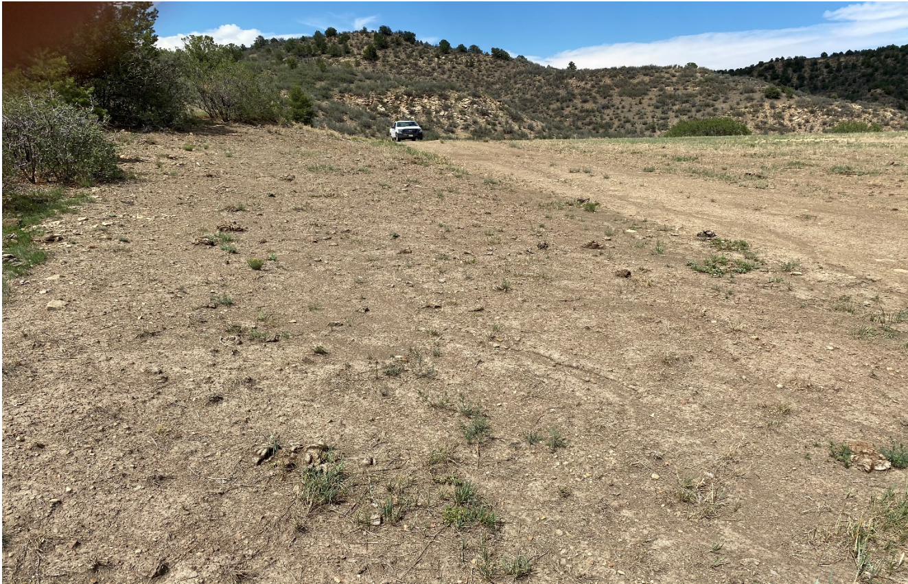
Photo 5. Facing north along the cut slope. Vegetation has not adequately established along the cut slope.
