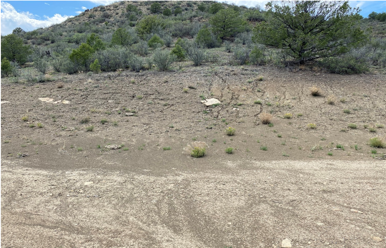
Photo 4. Facing toward the cut slope at the location. Vegetation has not adequately established and there are signs of erosion.
