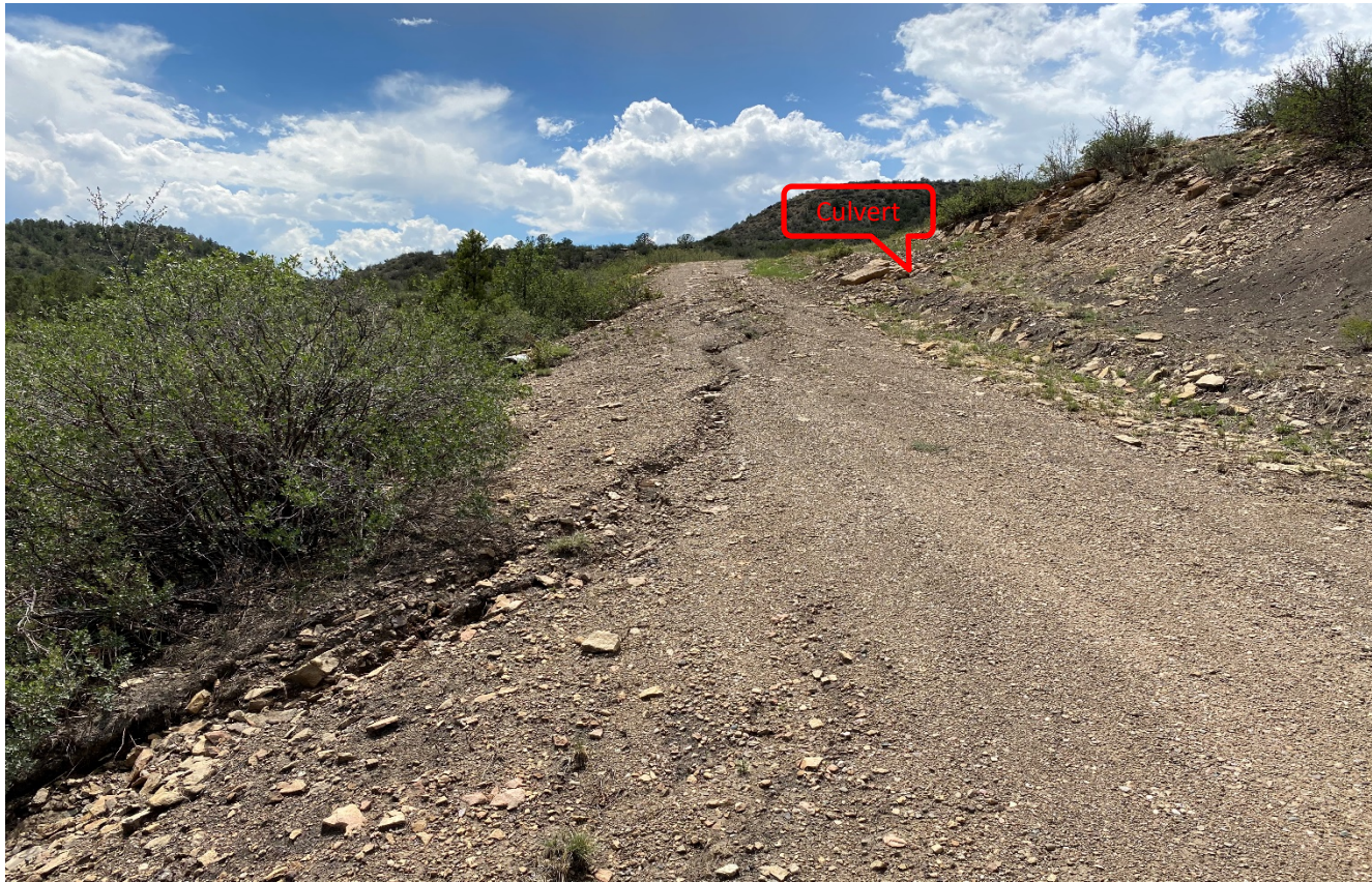
Photo 2. Facing west along the road ascending the hill. It appears stormwater is not properly directed toward the culvert causing erosion down the road.
