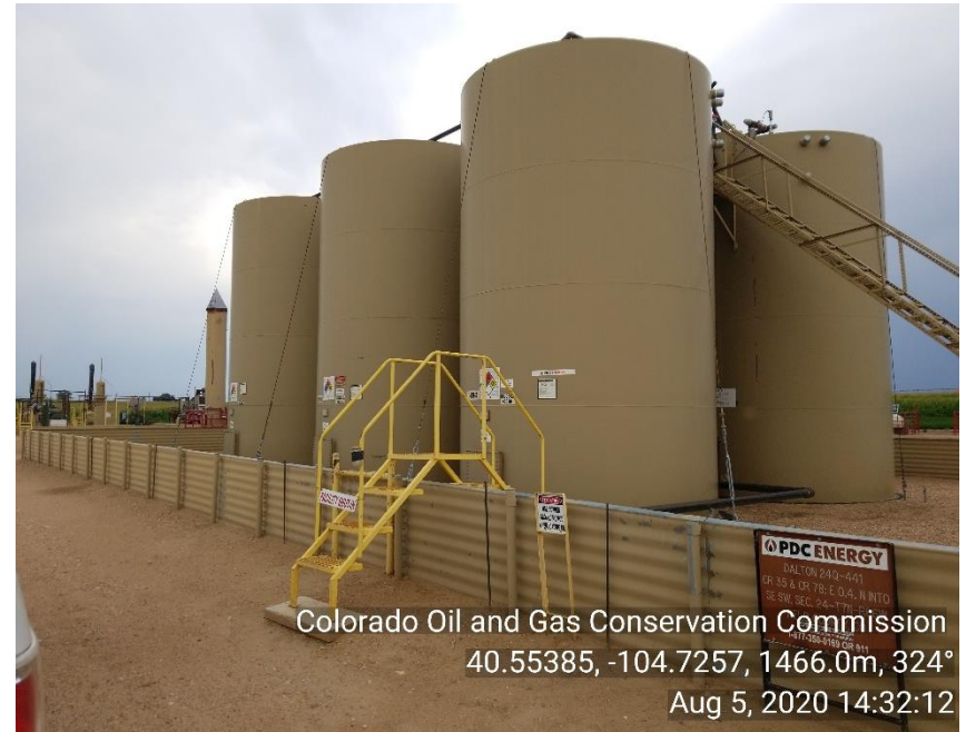
Photo 6: Tank Battery
