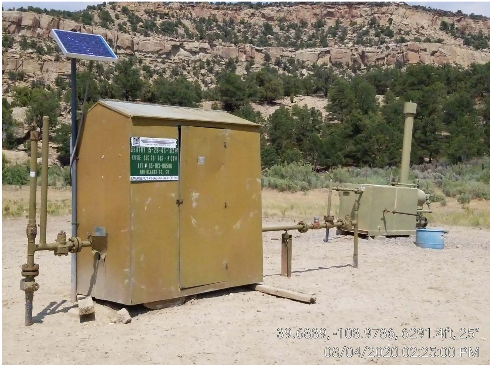
Photo 3. Meter building & separator.
