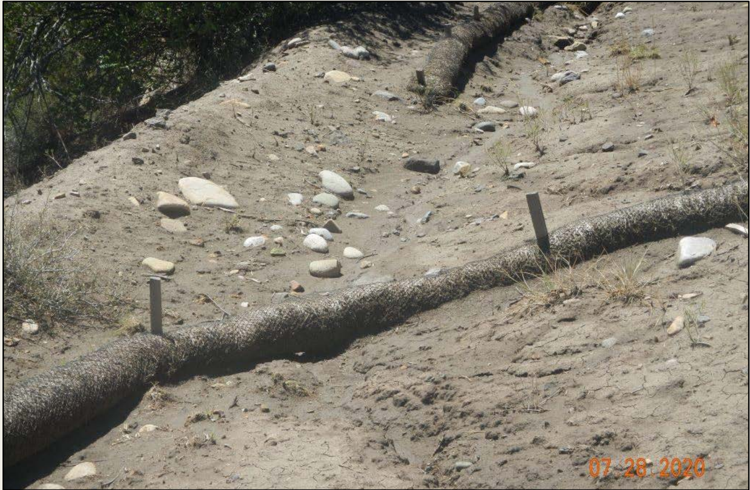
Photo 4. View of wattles in the southeastern project area that are no longer functioning and are not adequate BMPs in this area.
