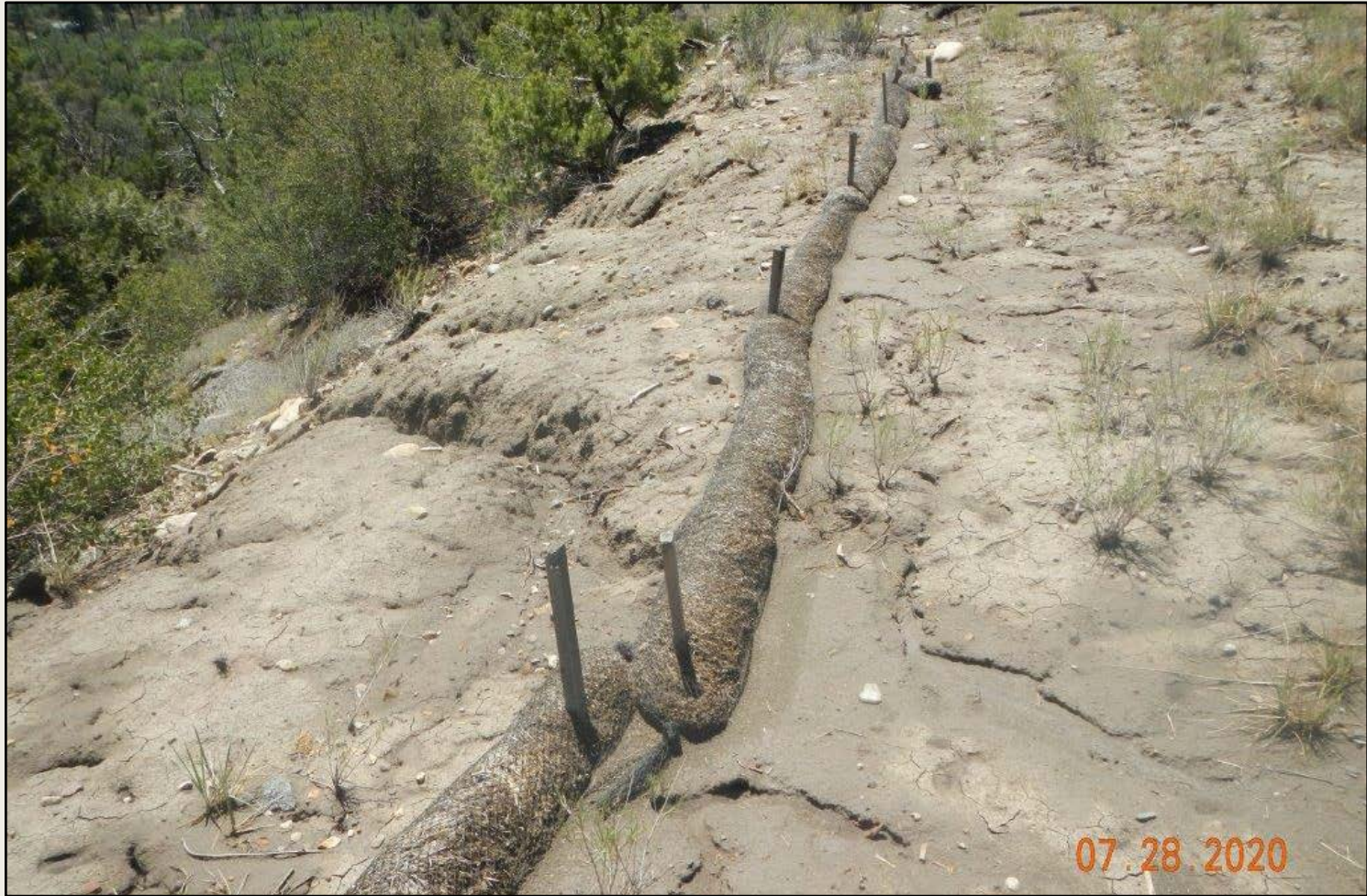
Photo 3. View of wattles along the eastern edge of the project area that are no longer functioning and are not adequate BMPs in this area.
