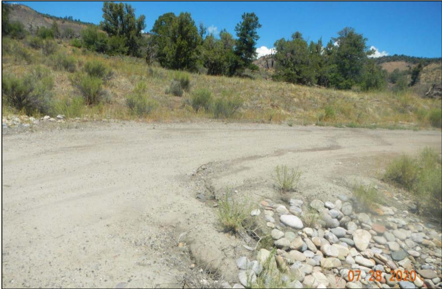
Photo 2. View of erosional channeling occurring at the well pad entrance where stormwater flows down the access road into culvert outlet (Photo 3).
