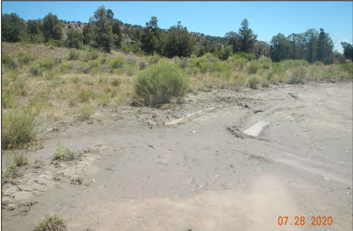
Photo 4. View of area along the well pad diversion, where diversion berm is damaged by truck tracks and erosion, and sediment is discharging onto the well pad resulting in deep rutting.
