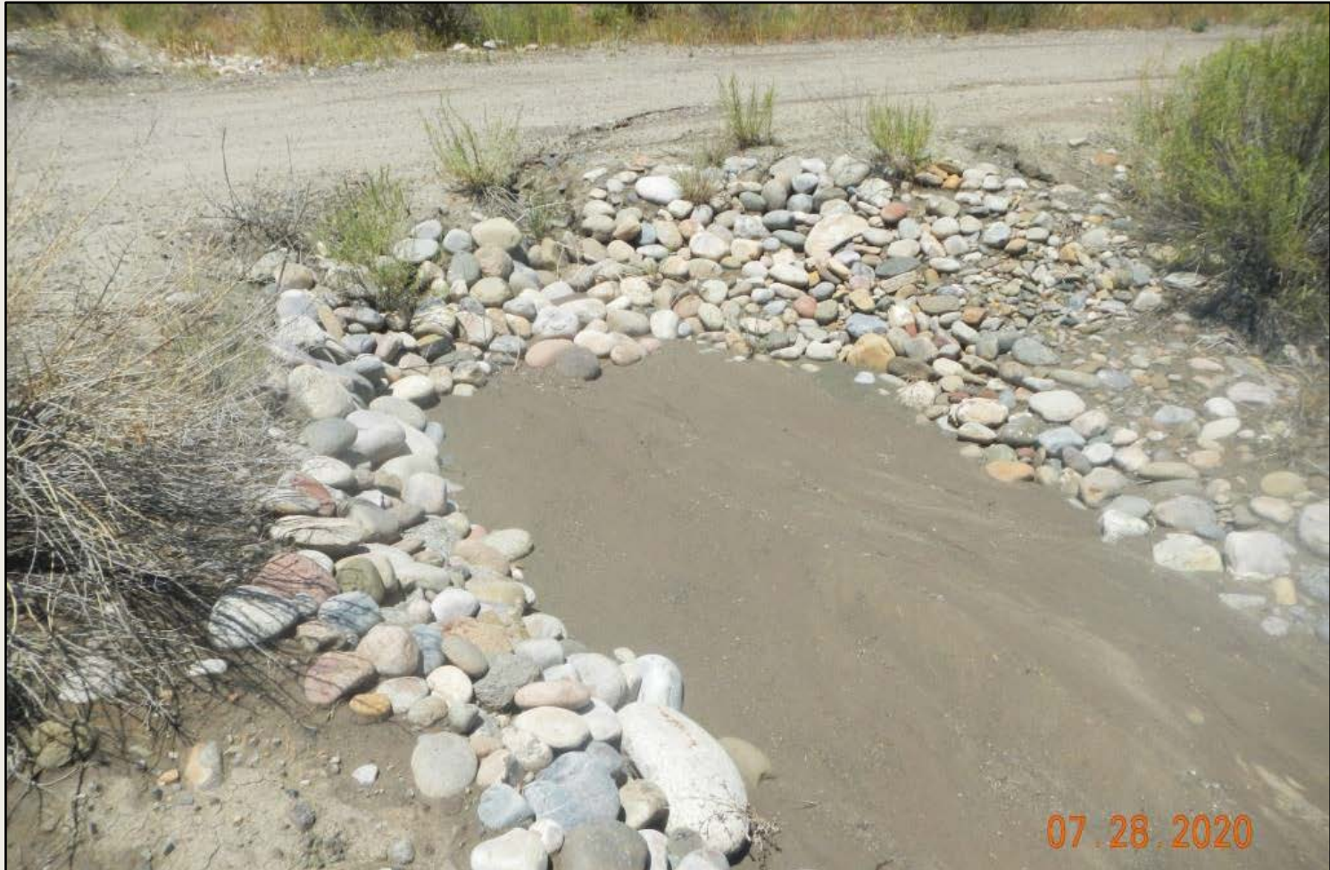
Photo 3. View of the culvert outlet at the well pad entrance. Culvert is full of sediment and needs maintenance.
