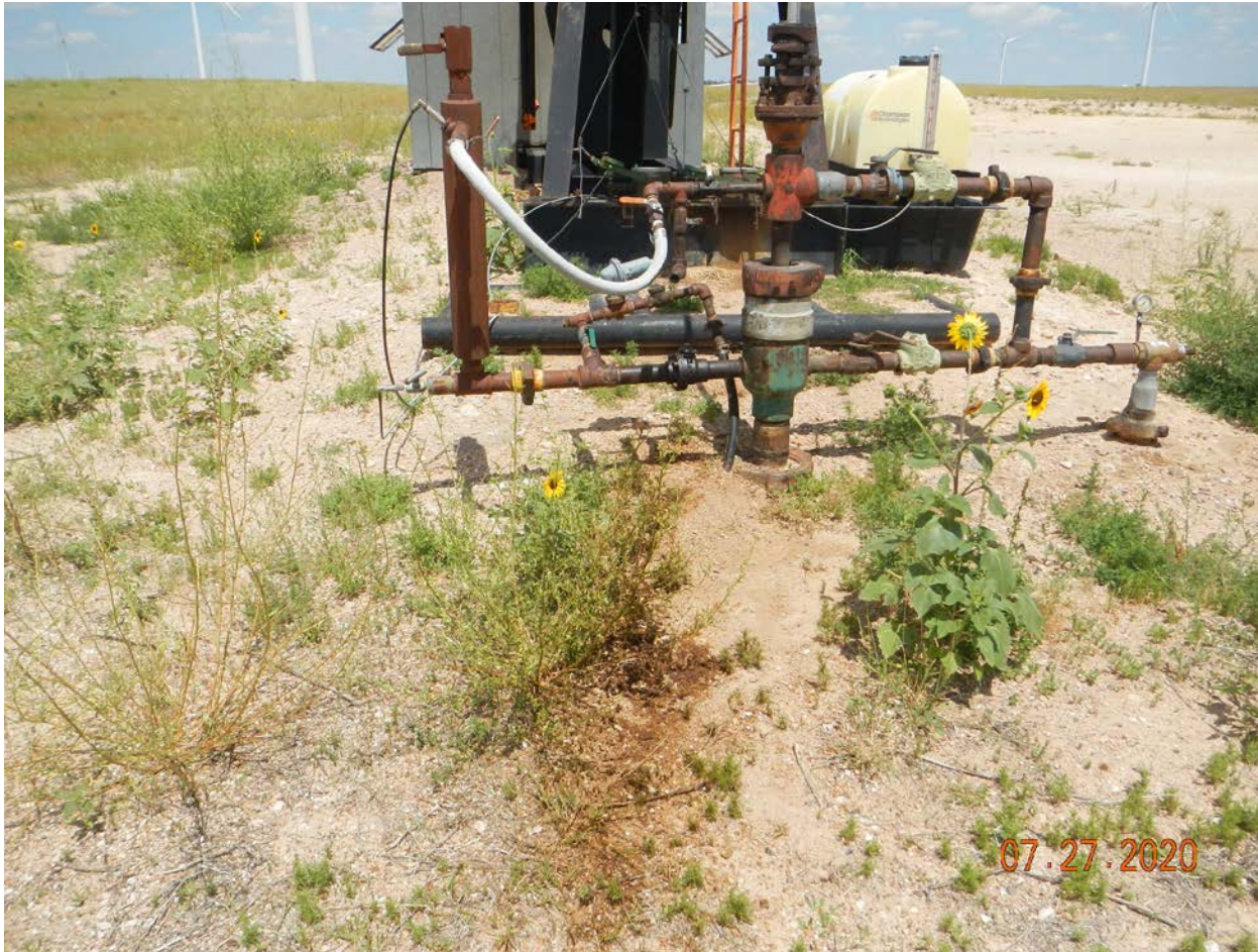
Photo # 6 – Oil stained soil related to wellhead valves
