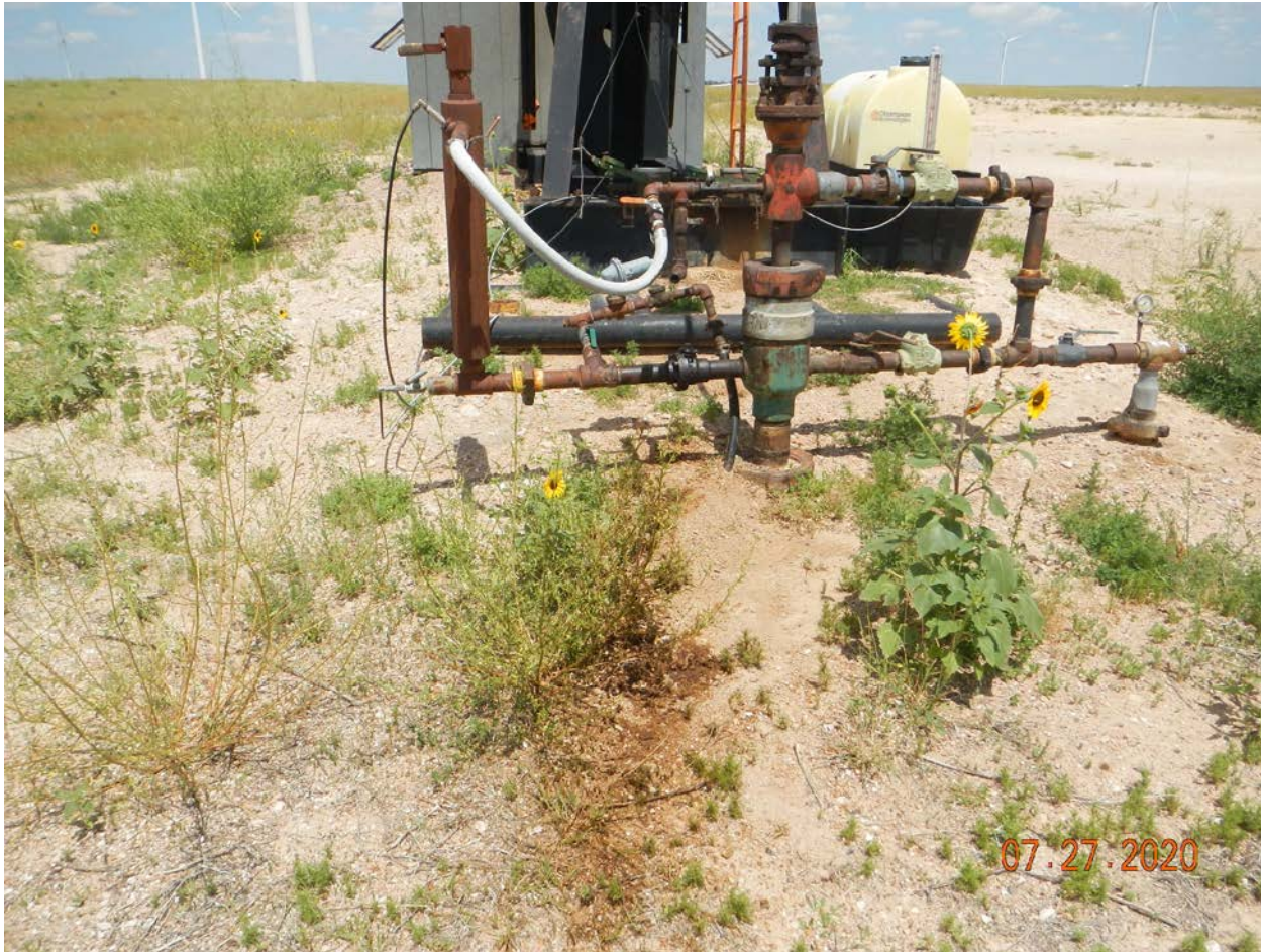
Photo # 5 – Oil stained soil related to wellhead valves
