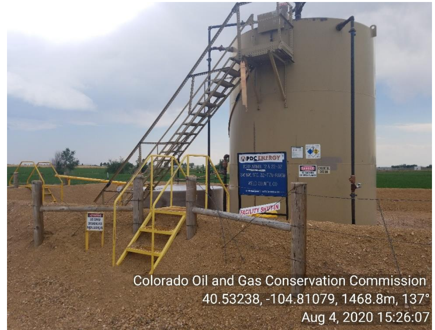
Photo 2: Tank Battery
