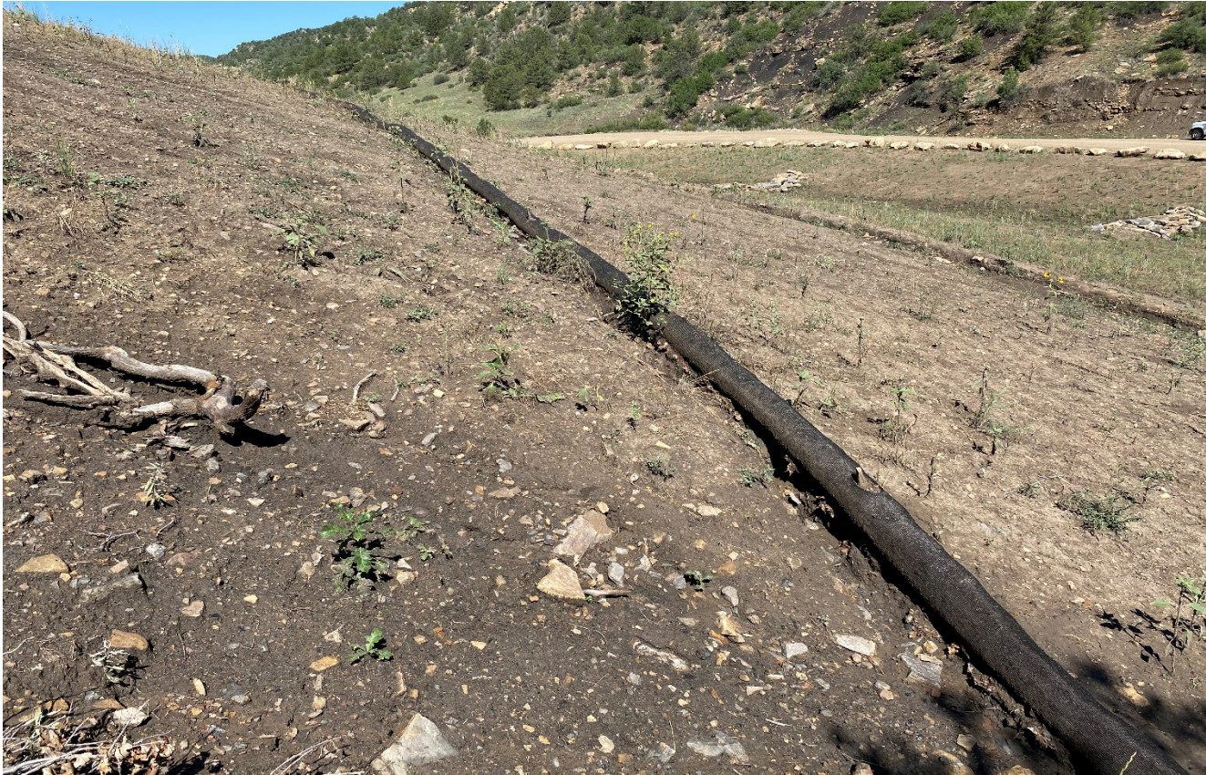
Photo 8. Facing northwest. The filtrex wattles appear to be working well but will need maintenance.
