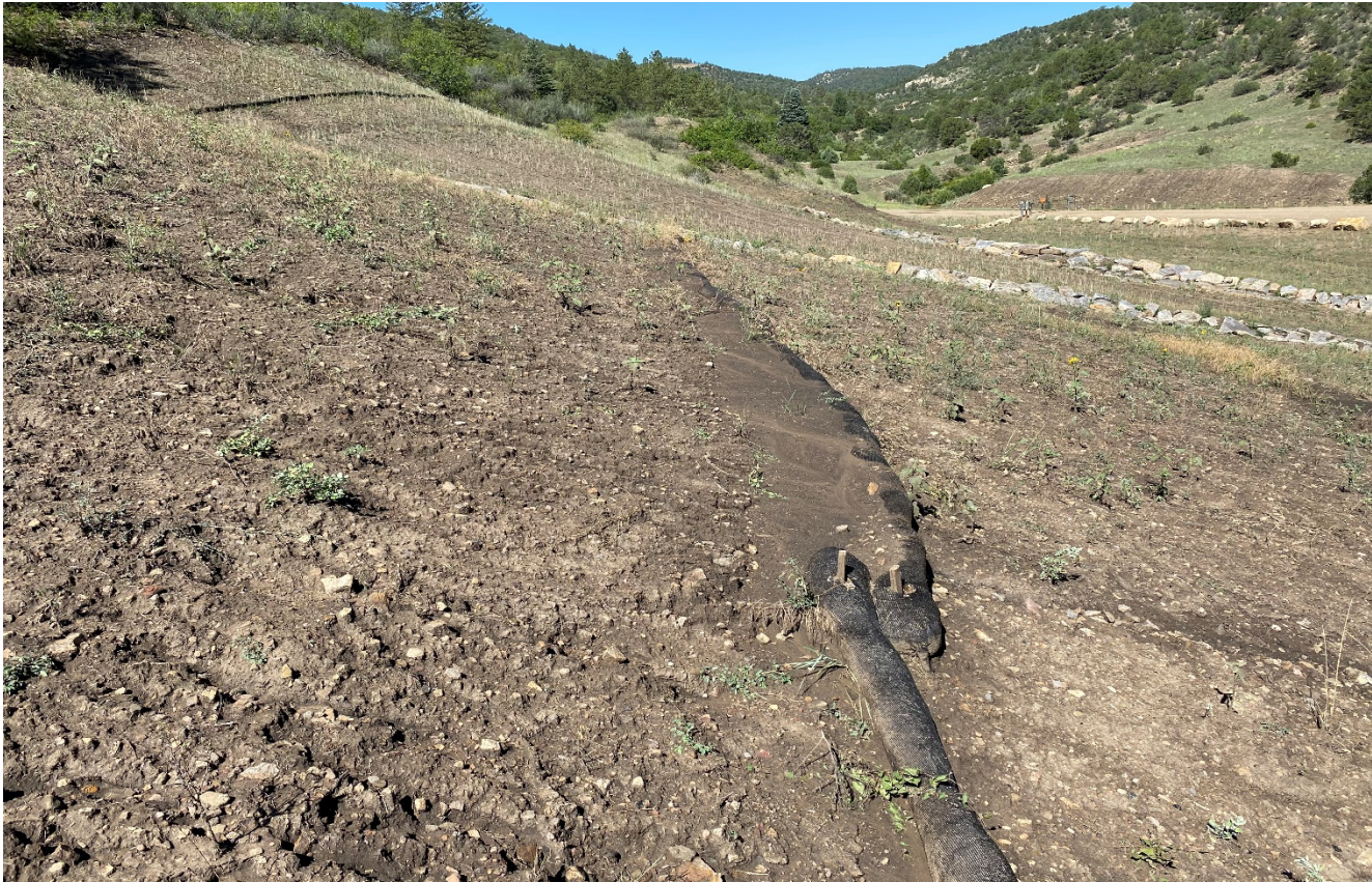
Photo 6. There are BMP's that have filled in with sediment and need maintenance.
