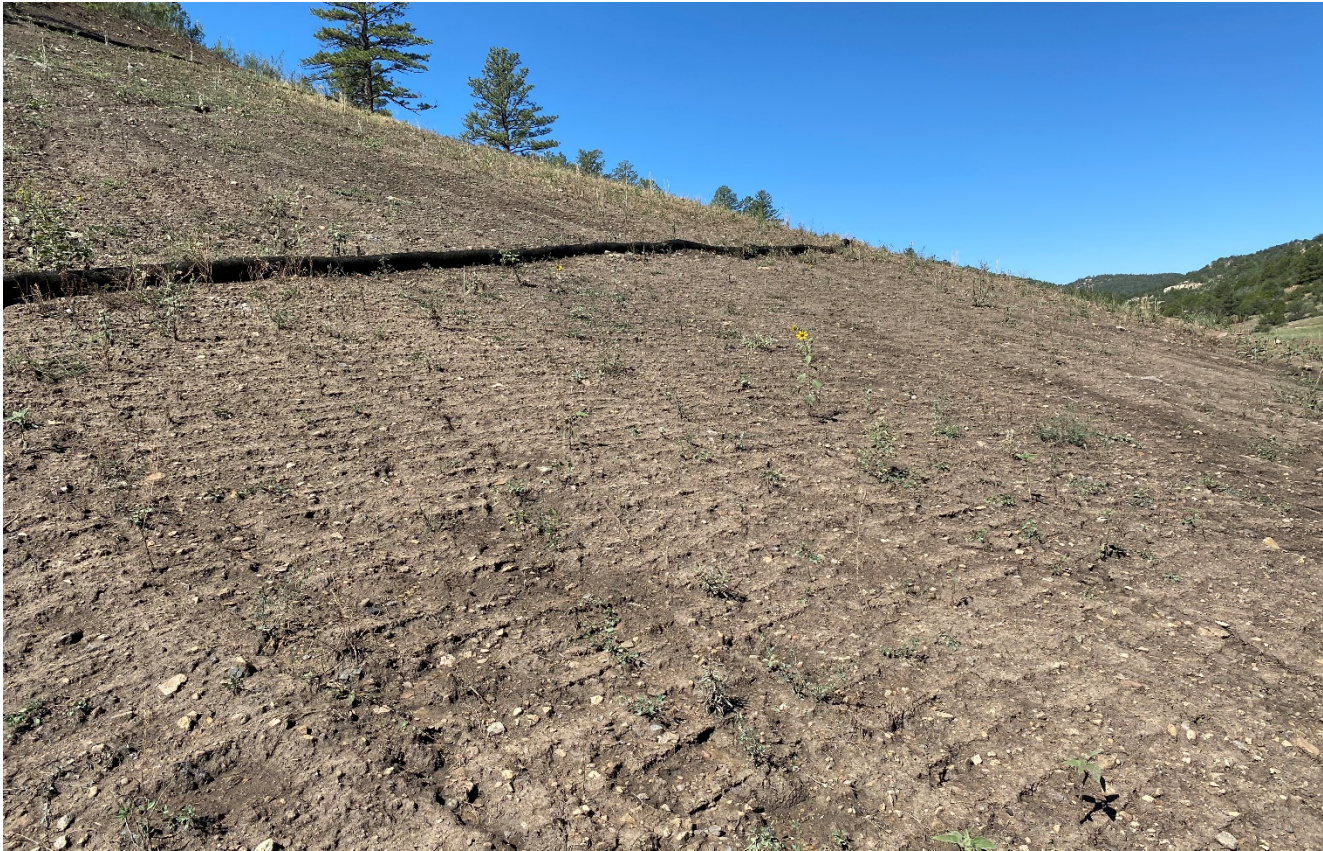
Photo 7. Facing toward the reclaimed slope. Vegetation does not appear to be establishing in areas of the location. Additional reseeding may be needed during the fall season.
