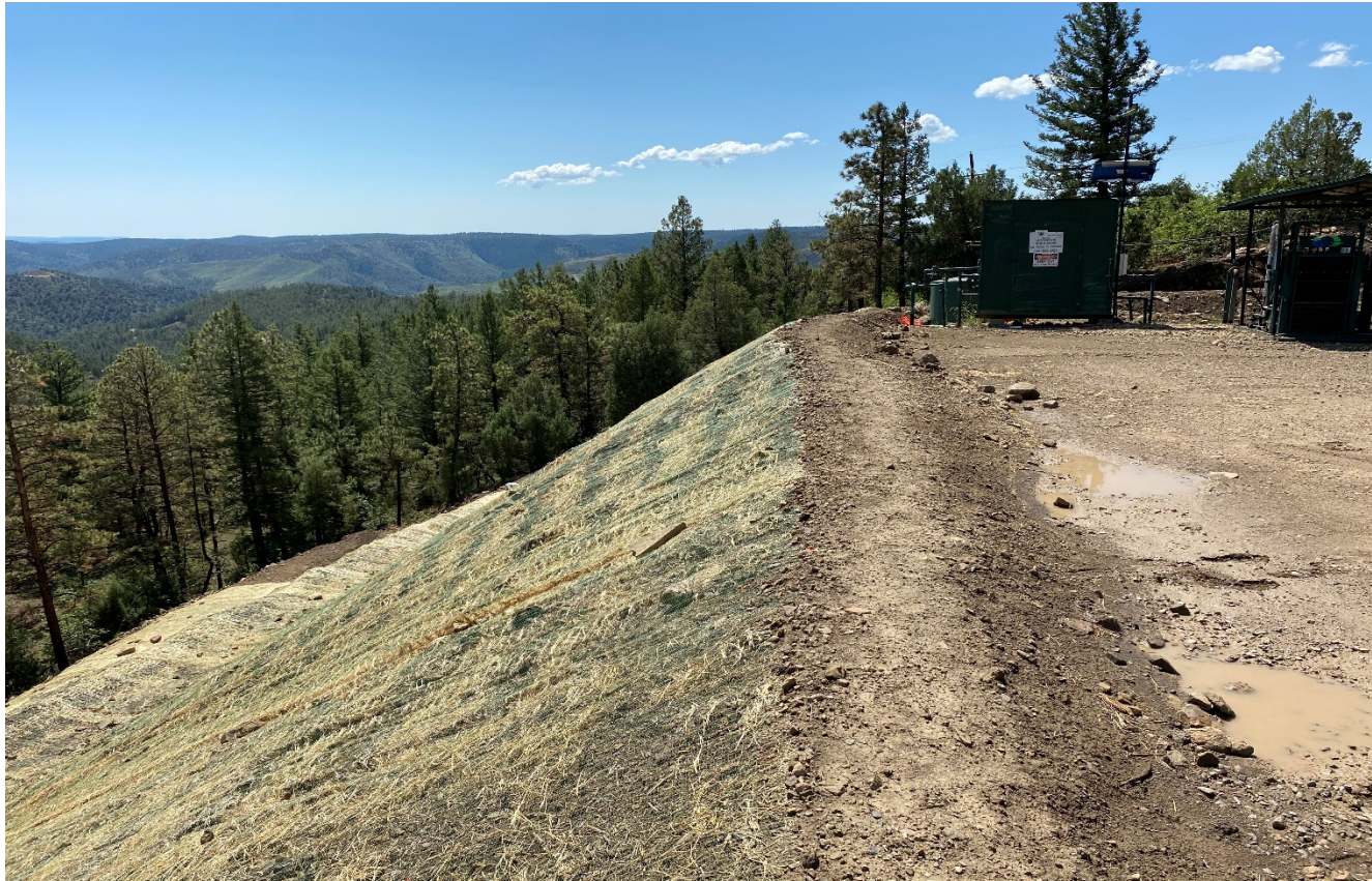
Photo 4. Facing southeast along the fill slope.
