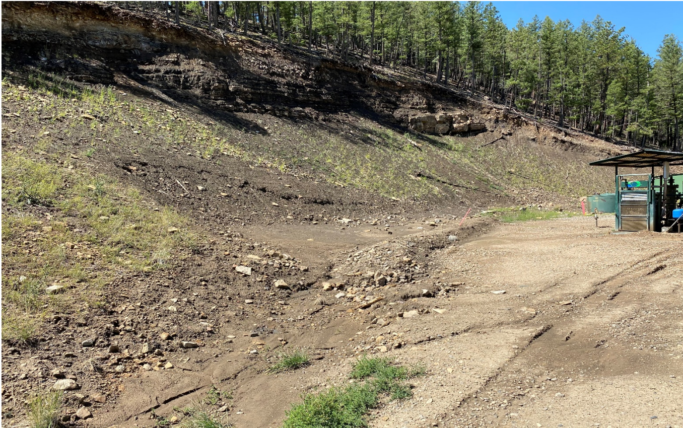
Photo 2. Facing southwest toward the cut slope of the location. Stormwater runoff from this area is causing erosion shown in previous photo. BMP's are needed in this area.
