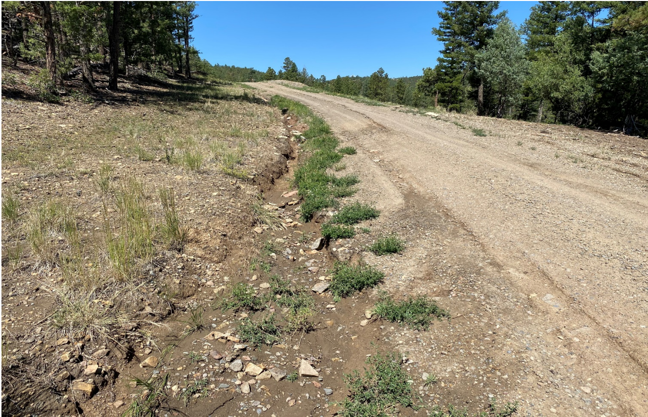
Photo 1. Facing west along the road near the location. Stormwater runoff from the location is directed down the road causing erosion. BMP's are needed in this area.
