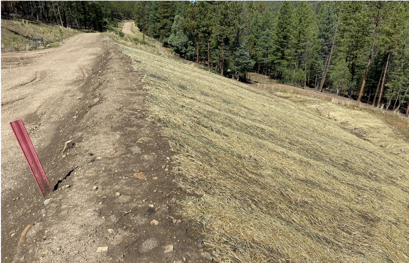
Photo 3. Facing northeast toward the fill slope. This area has been resloped and temporarily stabilized with straw blanket.
