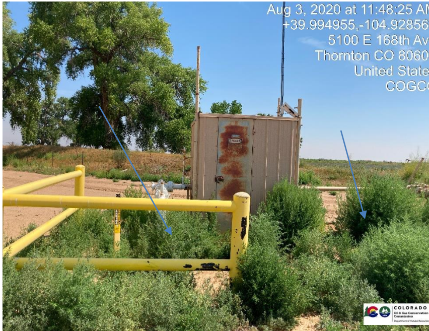
Pic 3 Unable to check calibration of gas meter run due to hornet nest inside/weeds around gas meter run
