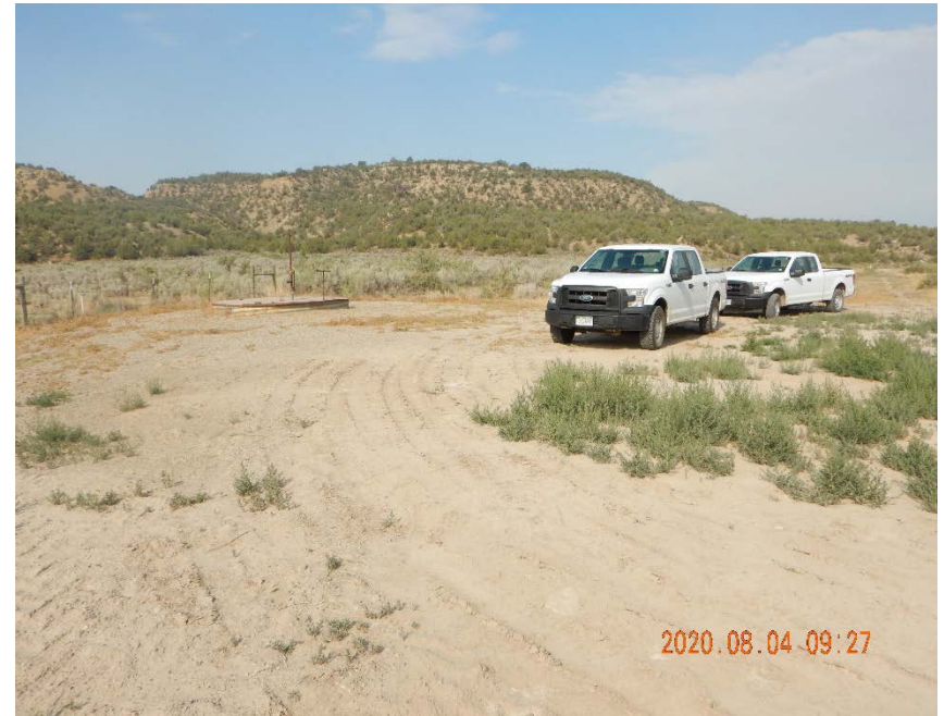
Photo #2 - View of valve can area, looking west.
