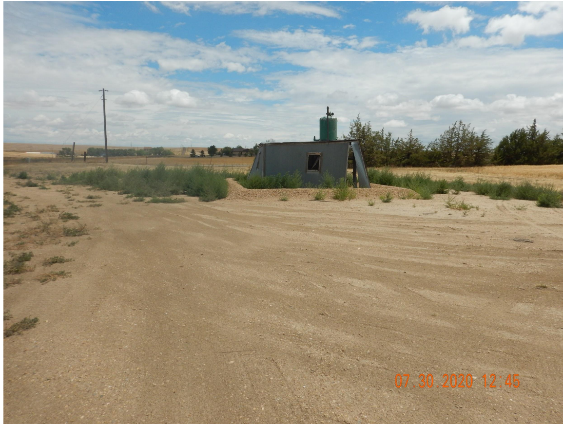
Photo 3. Photo taken from the tank battery, facing East. See comments under Photo 2.
