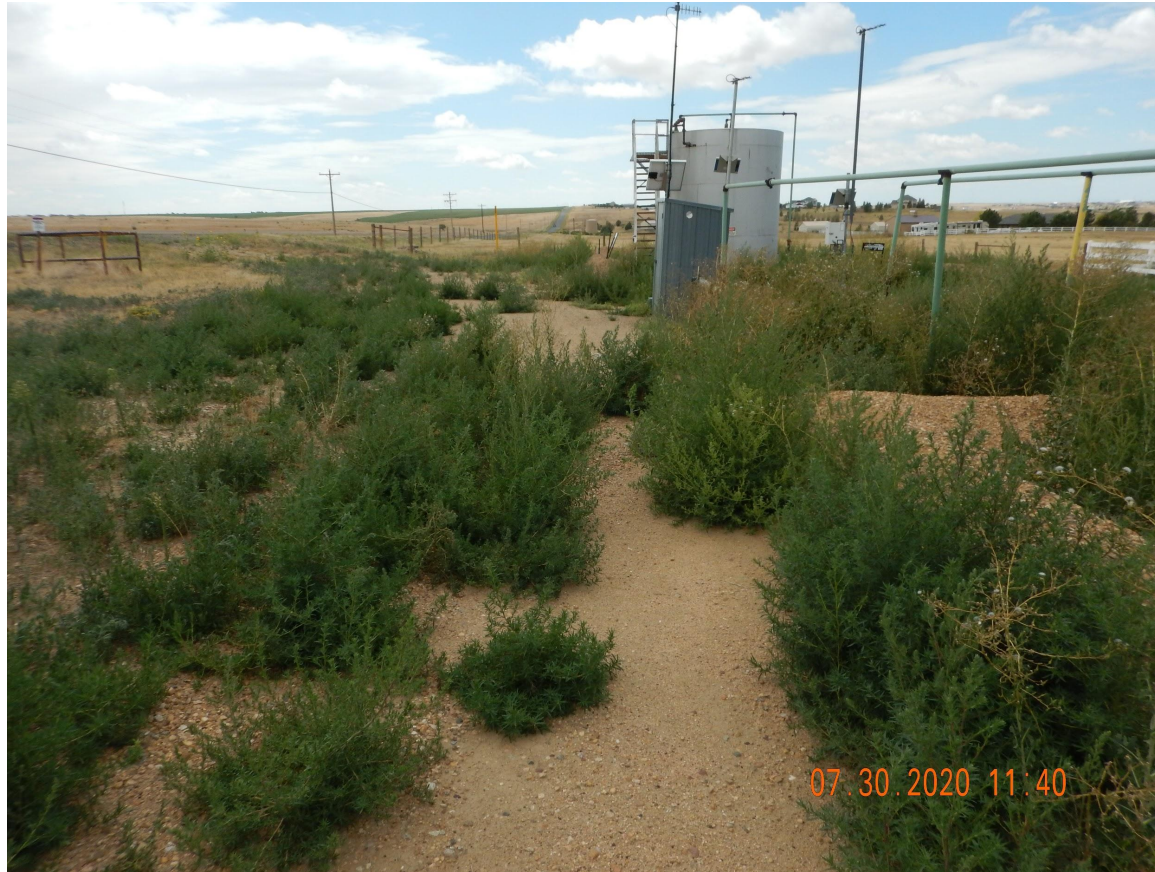
Photo 5. Photo taken from the central tank battery, facing South. See comments under Photo 3.
