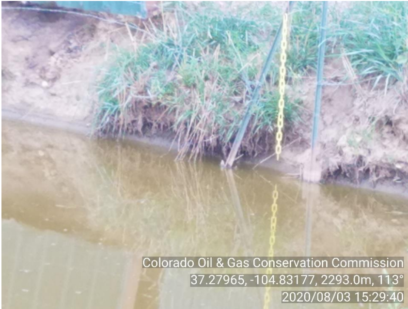
PHOTO 3: CA FOR FLUID LEVEL ABOVE FREEBOARD MARKER THAT WAS LISTED ON PREVIOUS INSPECTION HAS BEEN ADDRESSED. DOC#690200137
