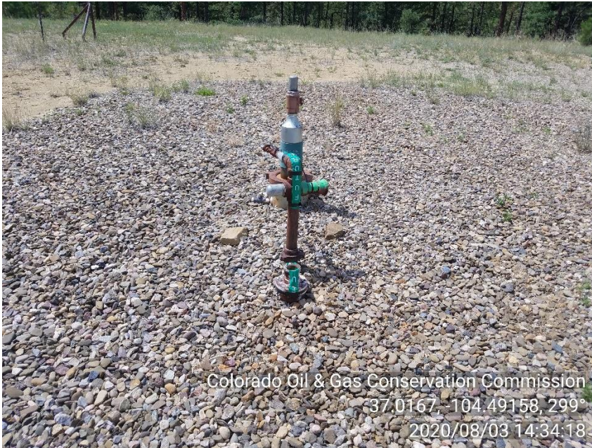
PHOTO 3: UNUSED RISERS NEAR WEST WELLHEAD NOT MARKED AS TO WHAT ITS USED FOR AND NO LO/TO. REMOVE OR PROPERLY MARK AND LO/TO PER RULE 603.f. CA DATE 11-3-20.
