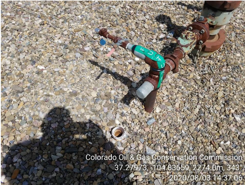
PHOTO 5: UNUSED RISERS NEAR EAST WELLHEAD NOT MARKED AS TO WHAT ITS USED FOR AND NO LO/TO. REMOVE OR PROPERLY MARK AND LO/TO PER RULE 603.f. CA DATE 11-3-20.
