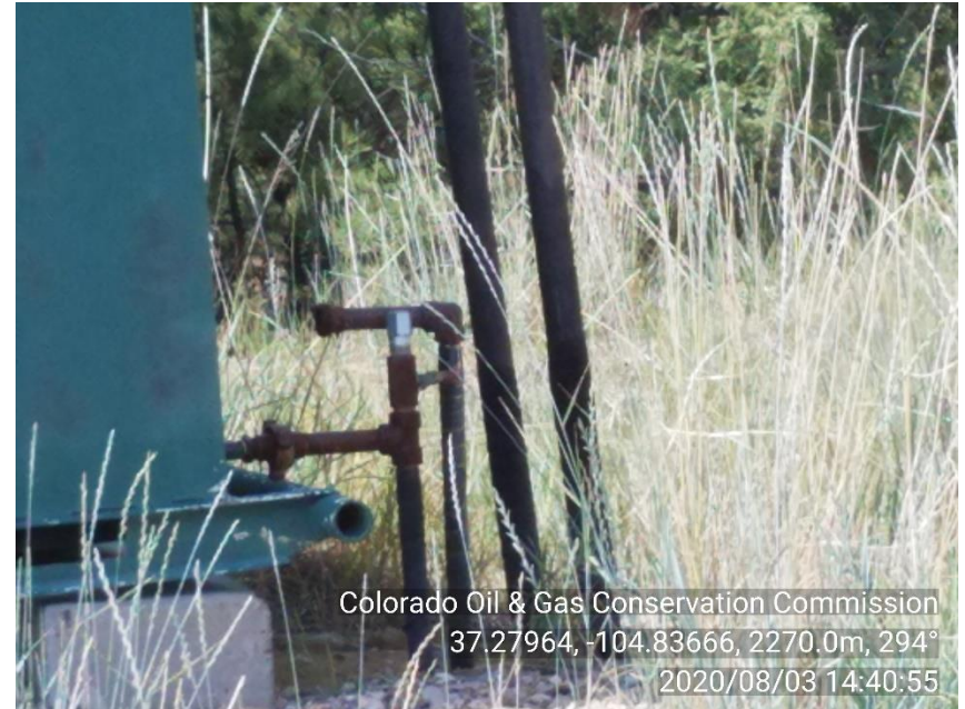
PHOTO 6: UNUSED RISERS NEAR METER HOUSE NOT MARKED AS TO WHAT ITS USED FOR AND NO LO/TO. REMOVE OR PROPERLY MARK AND LO/TO PER RULE 603.f. CA DATE 11-3-20.
