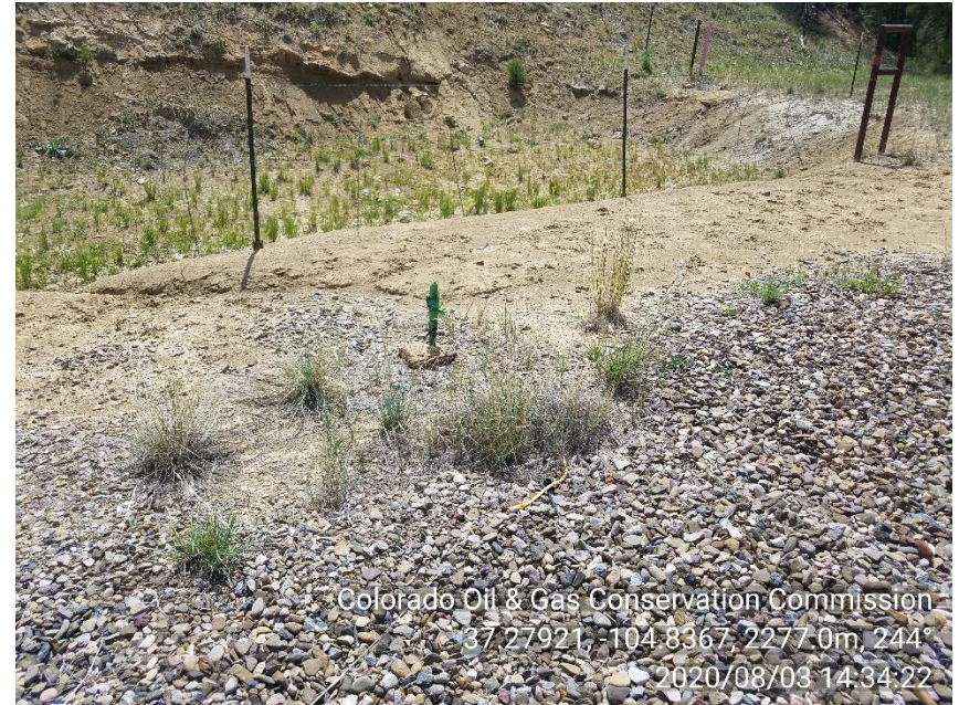
PHOTO 4: UNUSED RISERS NEAR WEST WELLHEAD NOT MARKED AS TO WHAT ITS USED FOR AND NO LO/TO. REMOVE OR PROPERLY MARK AND LO/TO PER RULE 603.f. CA DATE 11-3-20.
