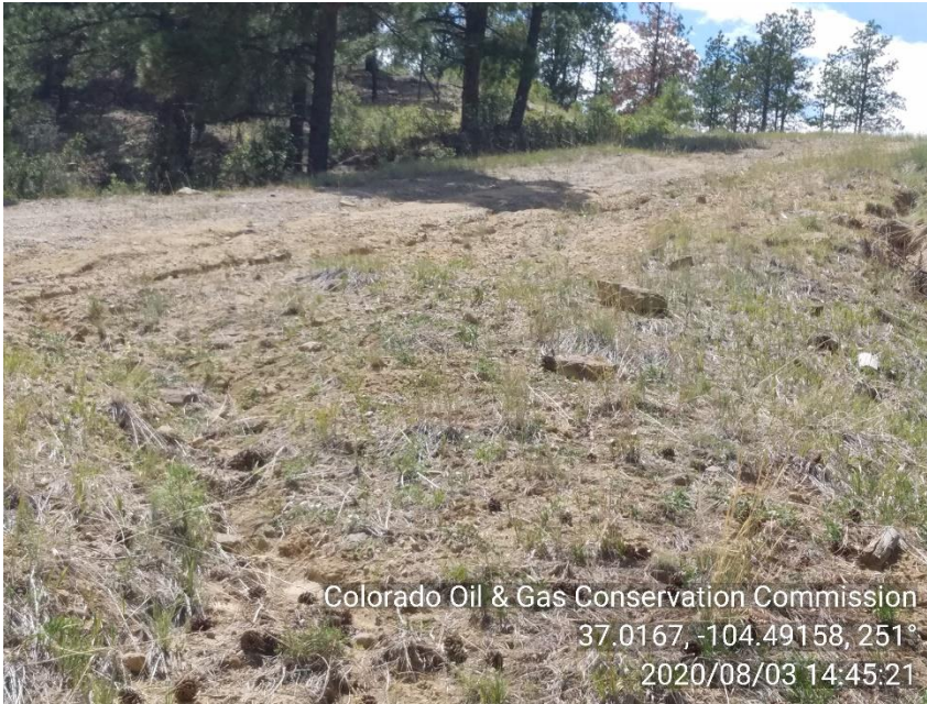
PHOTO 9: BMP'S ON ACCESS ROAD ARE FAILING AND OR IMPROPERLY INSTALLED. REPAIR AND INSTALL BMP'S TO CONTROL STORMWATER AND SEDIMENT FROM WASH DOWN ROADWAY PER RULE 1002.f.(2)C. CA DATE 11-3-20.
