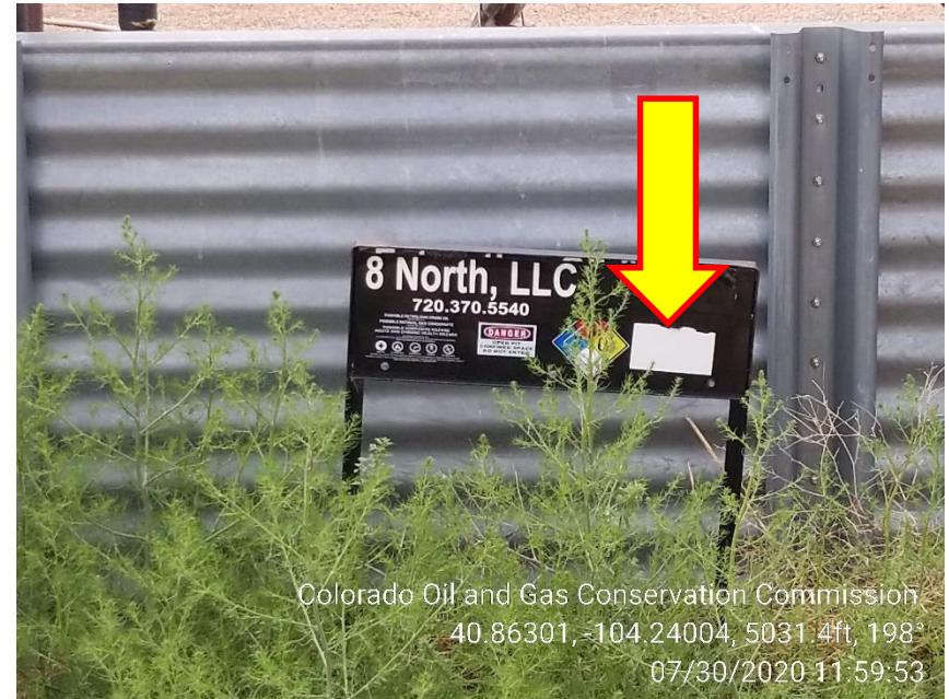
Photo 6 – Produced Water Tank missing Capacity Label
