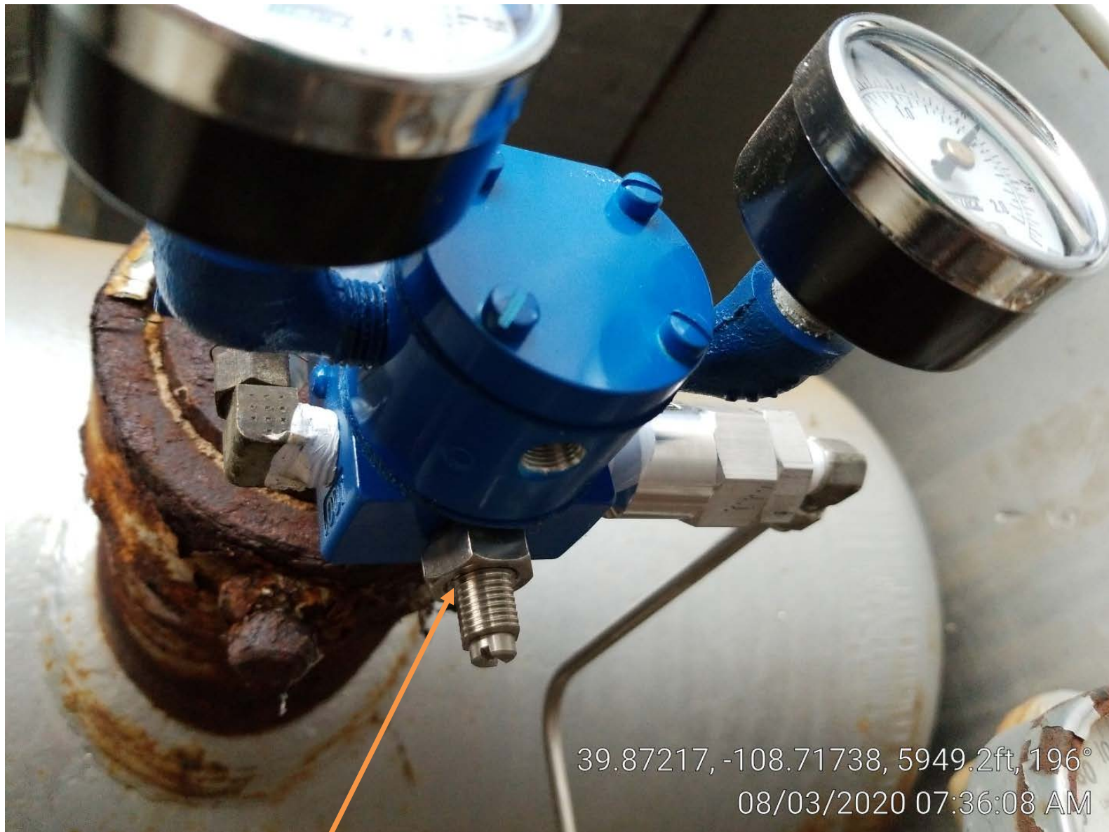
Photo 4. Gas leak at separator loose nut.
