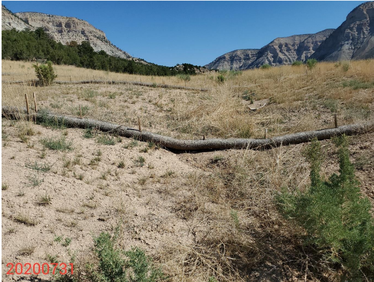
Photo 6: Photo taken from the south end of the Location, facing north. Photo shows wattle BMPs on Location have not been installed in accordance with good engineering practices; BMPs were placed/staked upon the soil surface, and have not been trenched and backfilled; Wattle BMPs are not in proper functioning condition. Stormwater has cut under the wattles and erosion degradation is evident
