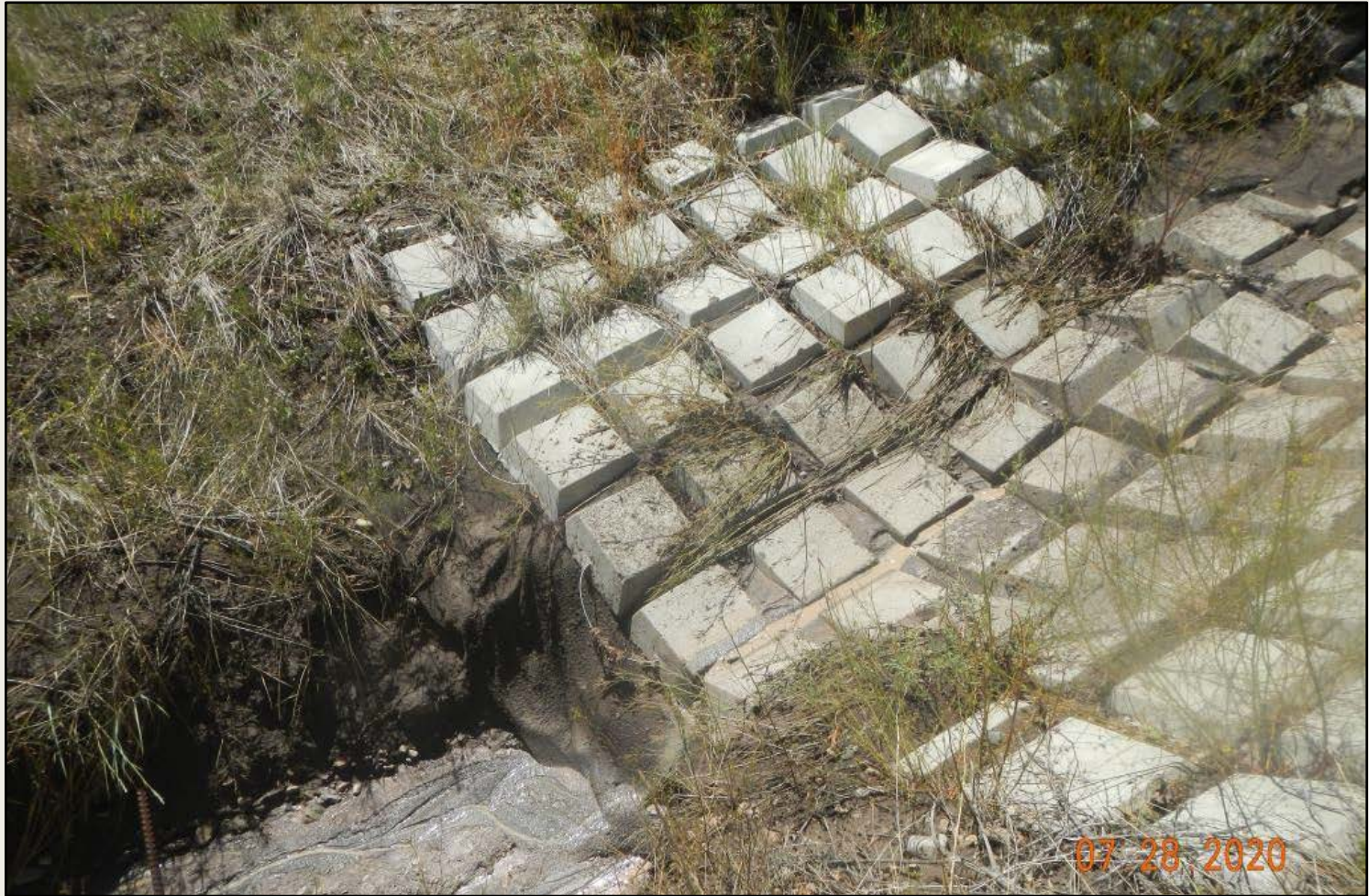
Photo 4. View of area at cement BMP, needing additional stabilization. Erosional downcutting is approximately 2.5 feet deep.
