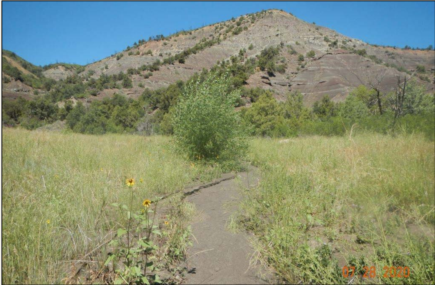
Photo 7. View of drainage channel that was re-connected at reclamation. Drainage elevation is approximately the same as up-stream elevation and appears to be functioning.
