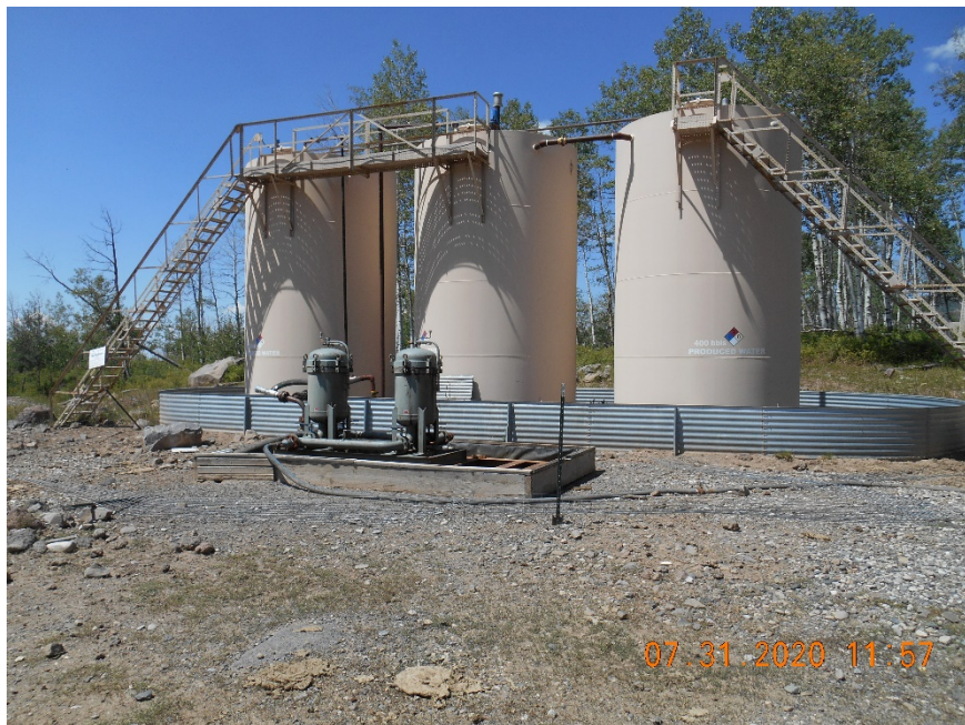
Tank battery and filter housings inside secondary containment.
