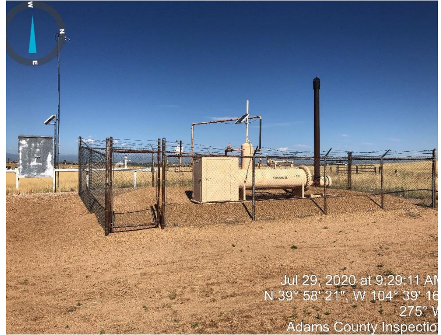
Photo #2 Meter and Separator.
