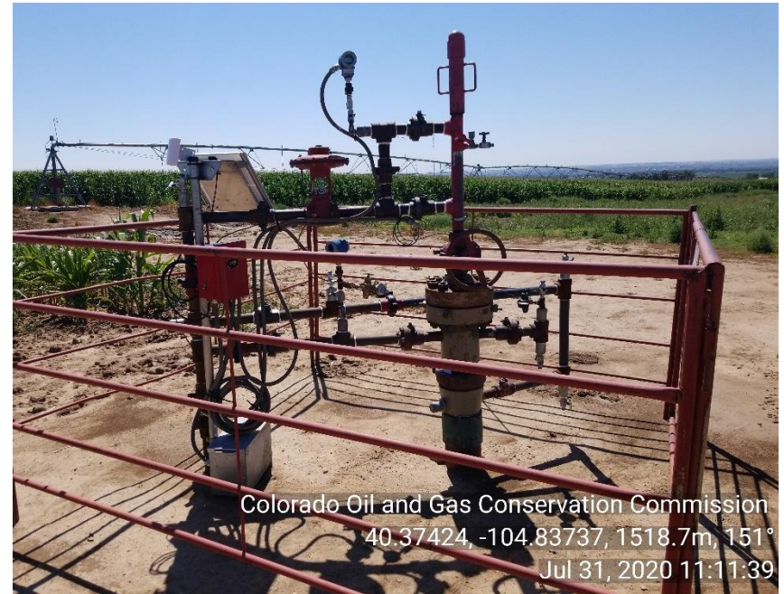
Photo 2: Wellhead; automation re-connected
