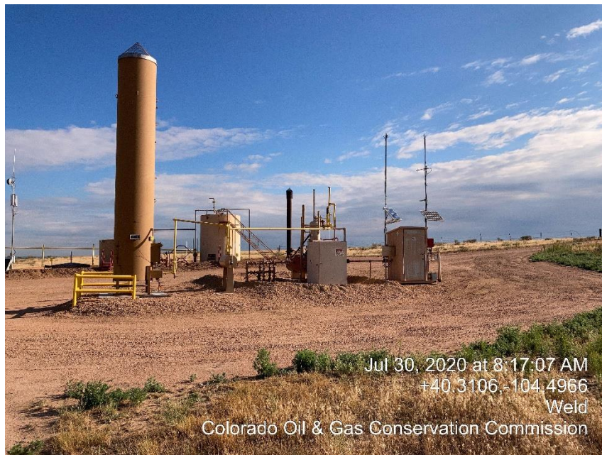
Photo #2 Separator, ECD & Meter Run
