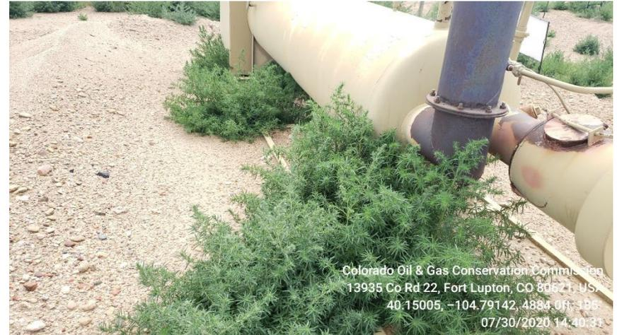
**Photo 5 weeds growing all around Horizontal Heated Separator**
