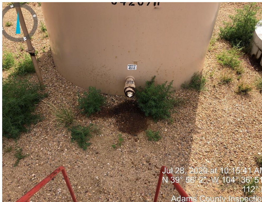
Photo #5 Stained soil next to Crude tank.
