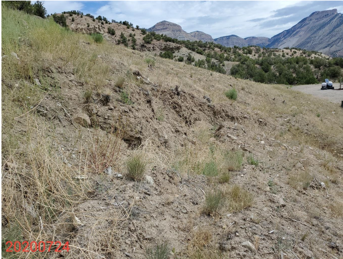
Photo 6: Photo taken from the southwestern interim areas, facing north. Photo shows erosion degradation on the slopes; Slopes do not appear to be sufficiently stabilized.
