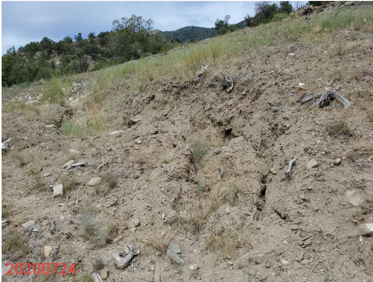
Photo 7: Photo taken from the southwestern interim areas, facing southwest. Photo shows erosion degradation on the slopes; Slopes do not appear to be sufficiently stabilized.
