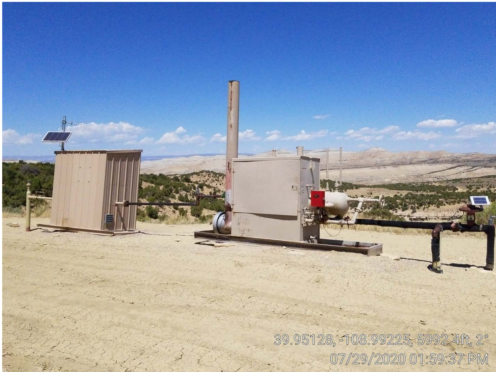
Photo 3. Meter building & separator.
