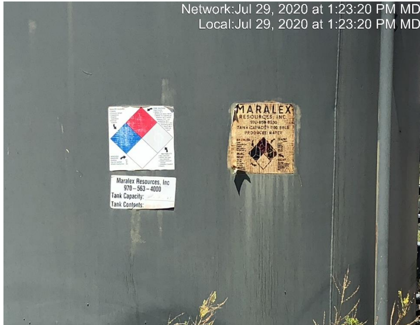
Photo #1640 Tank capacity, contents and NFPA label weathered and not legible.
