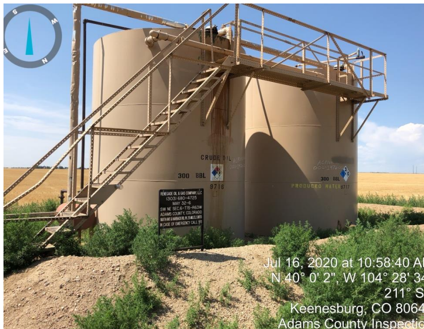
Photo#1 Production Tank and Produced Water Tank
