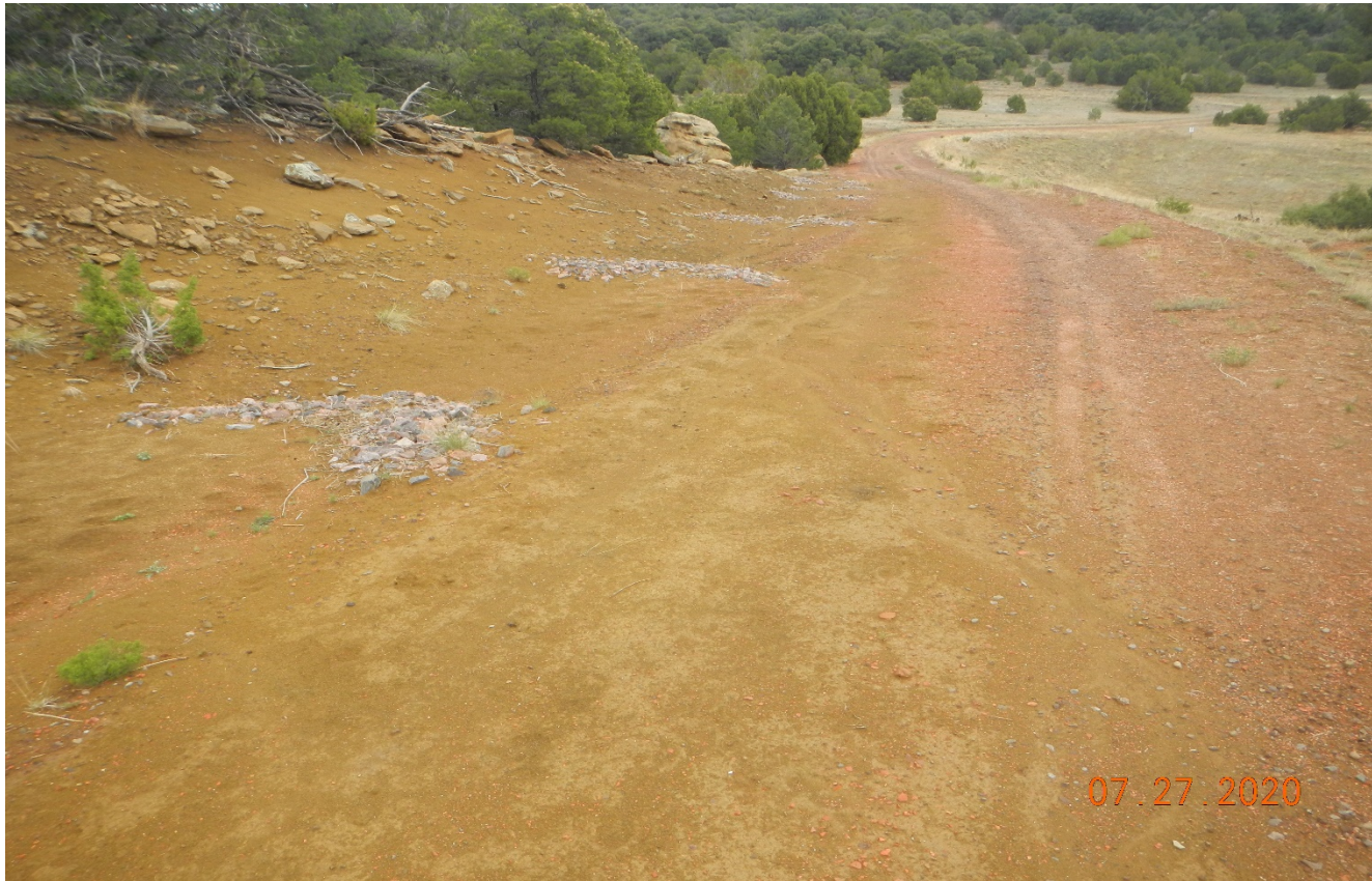
Photo 9. Facing southeast at the south side of the location. The access road continues toward the State 10WB. This check damn has filled in with sediment. The side of road needs to be seeded and stabilized.
