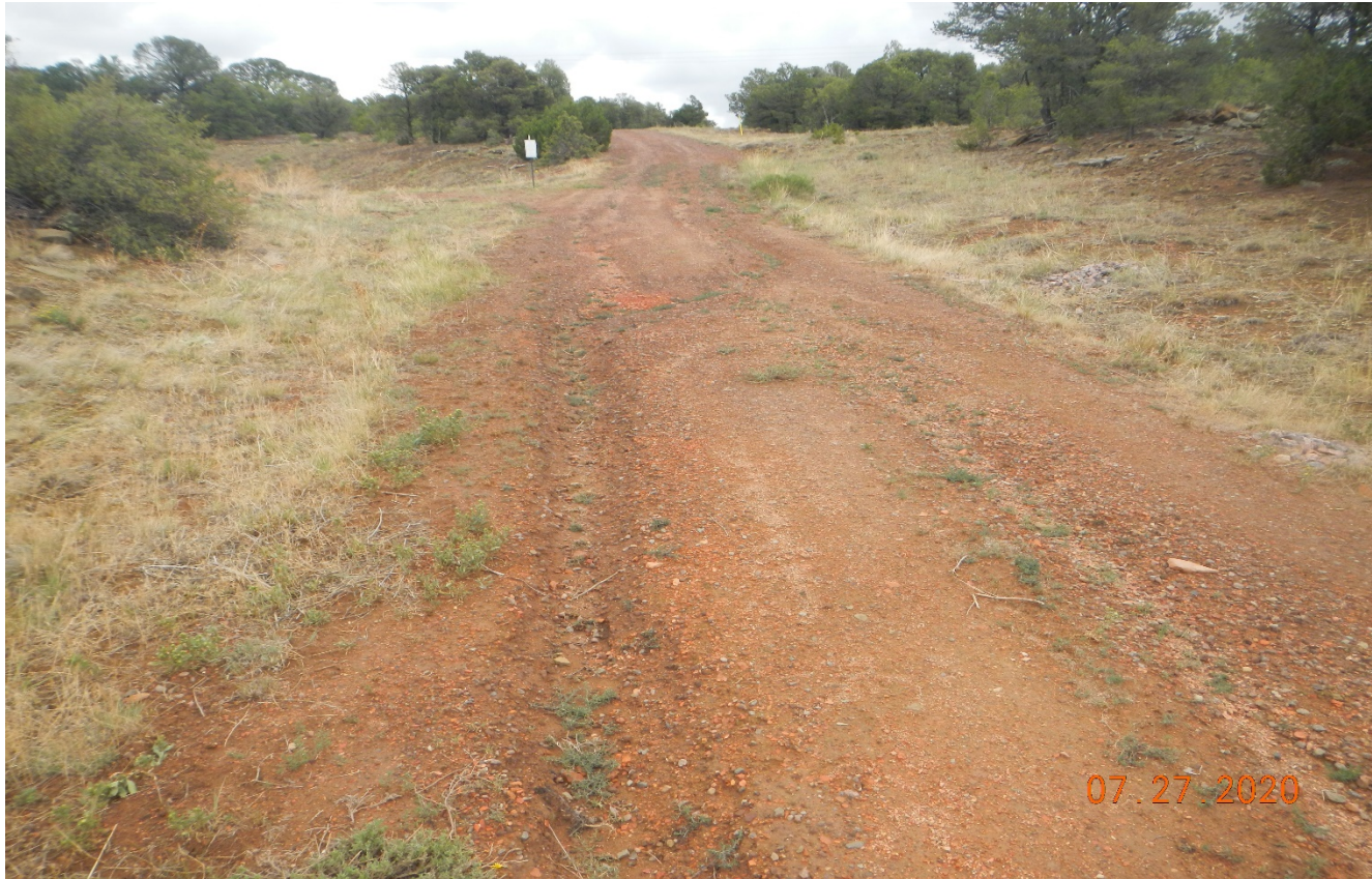
Photo 2. Signs of stormwater flowing down the road causing erosion near the State 7W location.
