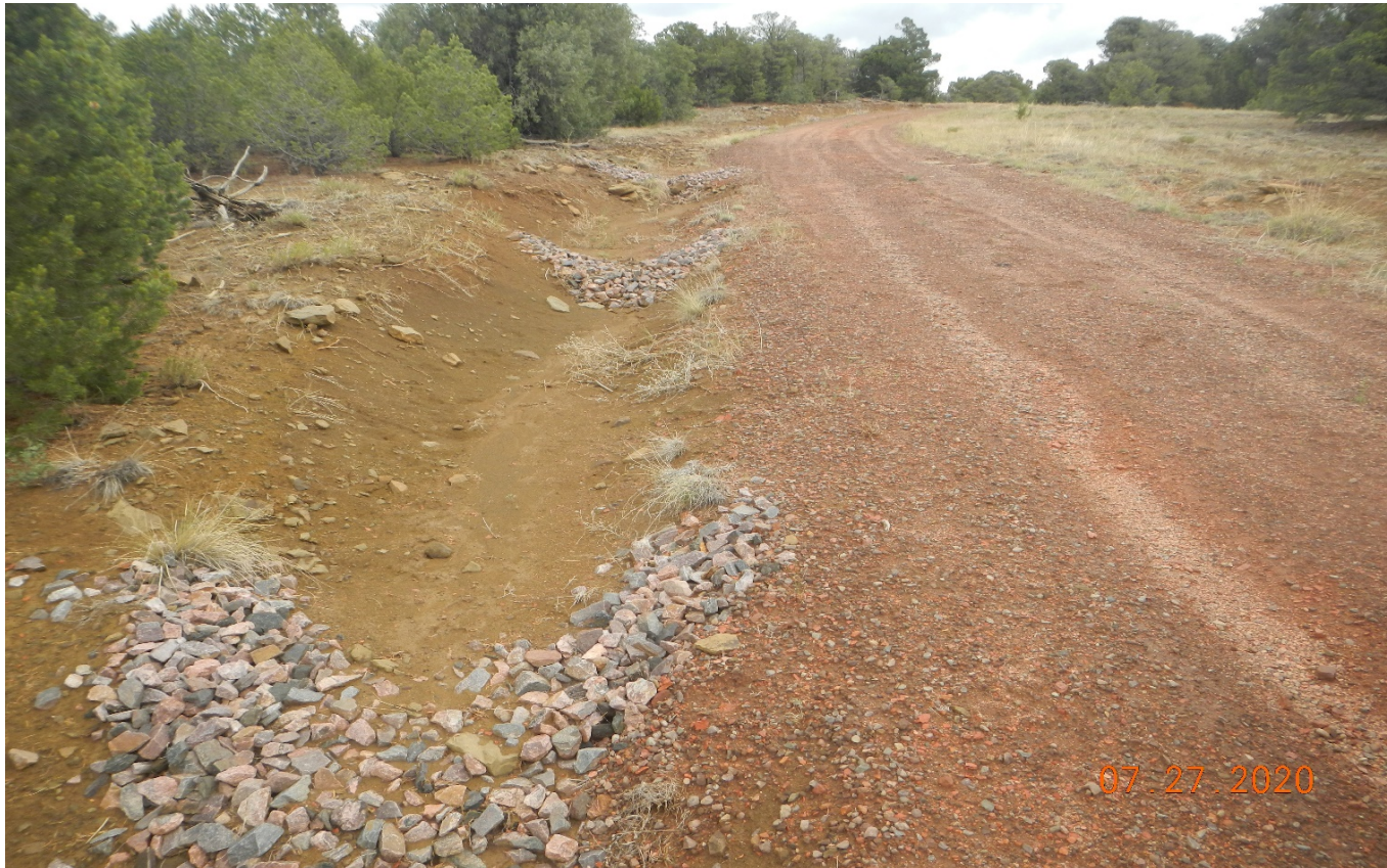
Photo 3. The check dams have filled in with sediment which are not maintained.
