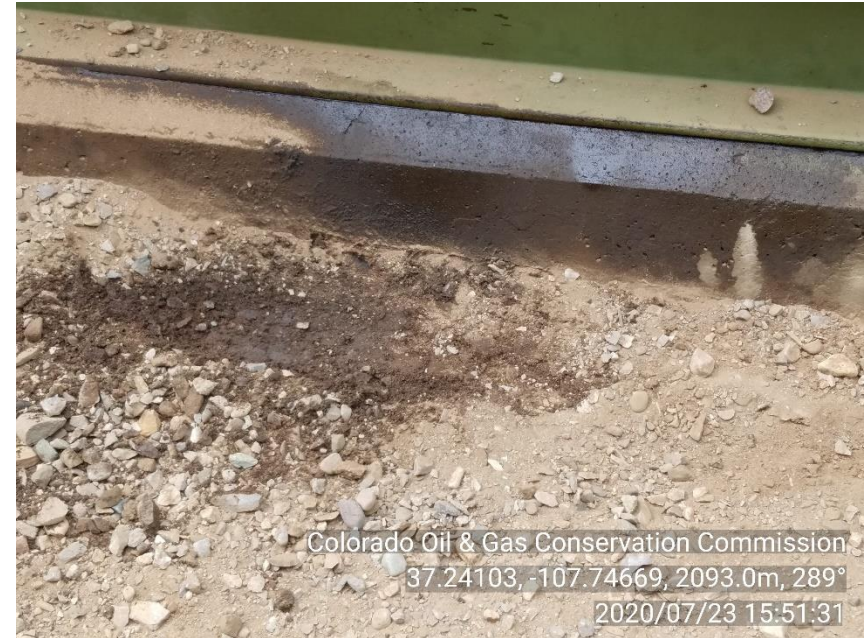
PHOTO 4: AFTER NOTICING WHAT APPEARS TO BE USED OIL RUNNING DOWN CONCRETE PUMPJACK PAD I KICKED FRESH LAID DIRT ASIDE AND REVEALED AN AREA OF IMPACTED SOIL ON GROUND NEXT TO PUMPJACK ENGINE. Conduct maintenance on equipment, cleanup stained material and review self inspection processes. CA DATE 10-23-20.
