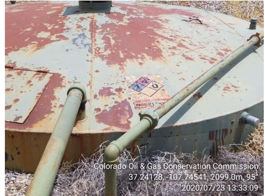
PHOTO 6: NFPA STICKER IS FAIDED AND ALMOST NOT LEGIBLE ALSO THERE IS NO TANK CAPACITY POSTED ON TANK. POST SIGNS IN COMPLIANCE WITH RULE 210.d ca date 10-23-20.
