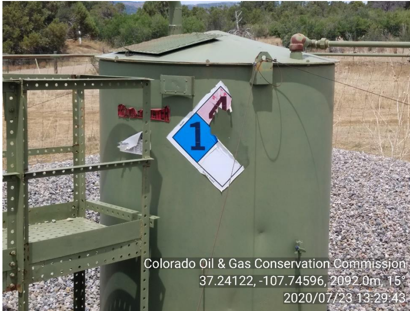
PHOTO 5: NFPA STICKER FAIDED AND FALLING APART. POST NFPA STICKERS IN COMPLIANCE WITH RULE 210.d. CA DATE 10-23-20.
