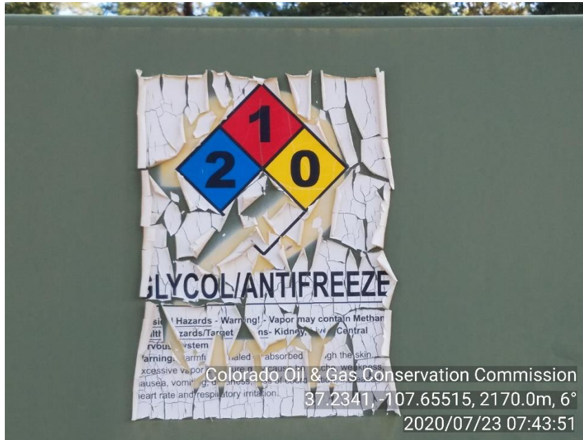
PHOTO 5: PLACARD ON SEPARATOR IN CRACKING AND STARTING TO FALL OFF. PLACARD WITH NEED REPLACED SOON.
