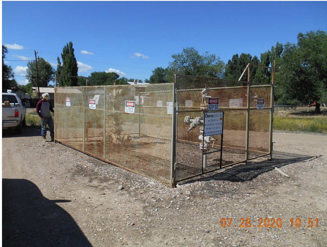
Injection wellhead – Temporarily abandoned
