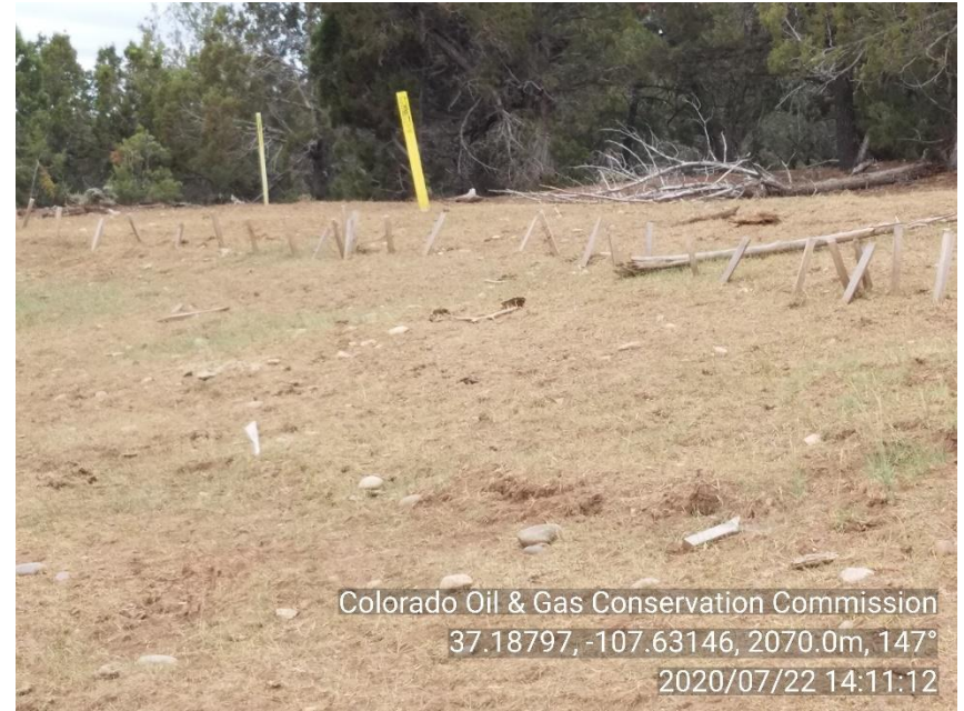
PHOTO 8: UNUSED EQUIPMENT (STAKES FOR WADDLES ARE LEFT ON INTERIM RECLAMATION AREA AROUND LOCATION). REMOVE UNUSED EQUIPMENT PER RULE 603.f. CA DATE 10-22-20.
