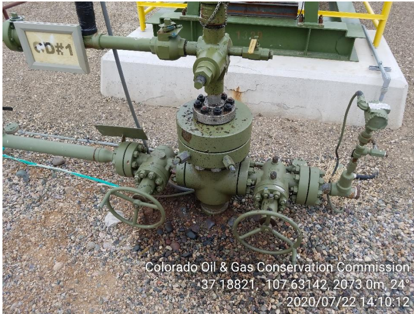
PHOTO 7: Approx 2' x 2' area of stained soil/gravel around base of STATE CD 3 wellhead. Clean-up and dispose of stained soil/gravel per Rule 1102.f.(2) and Rule 907.e. CA DATE 8-12-20.
