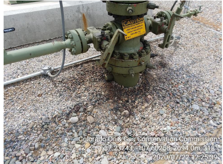
PHOTO 4: Approx 2' x 2' area of stained soil/gravel around base of wellhead. Clean-up and dispose of stained soil/gravel per Rule 1102.f.(2) and Rule 907.e. CA DATE IS ORIGINAL FROM PREVIOUS INSPECTION DOC#687904818
