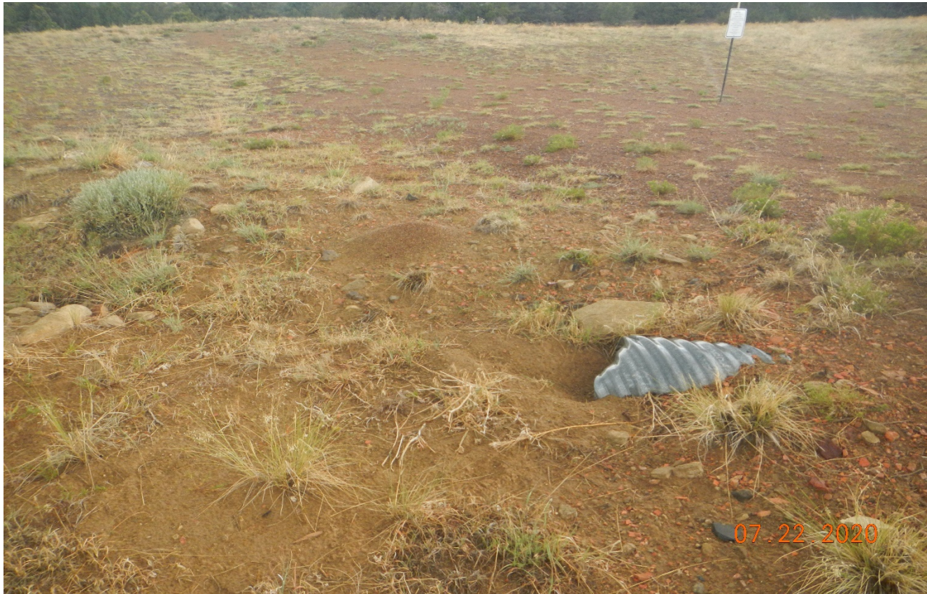
Photo 3. The outlet culvert has filled in with sediment and has not been maintained.
