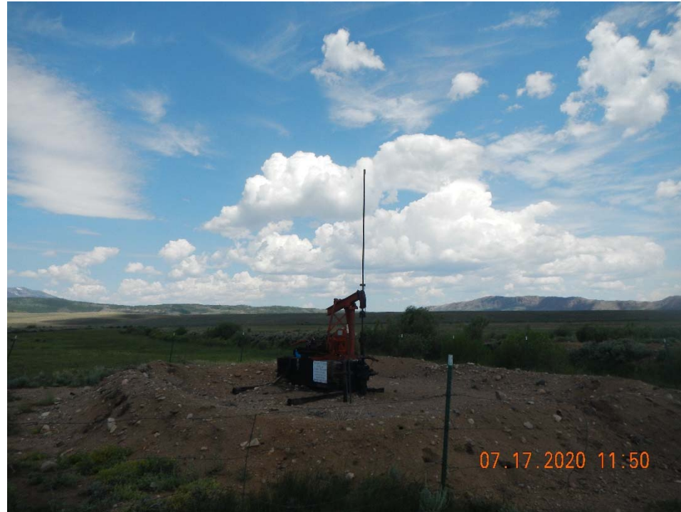
Photo 1. Overview of location taken facing north
