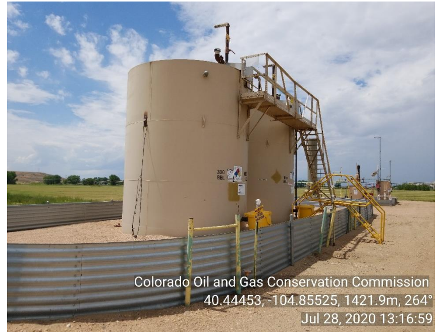
Photo 2: Tank Battery
