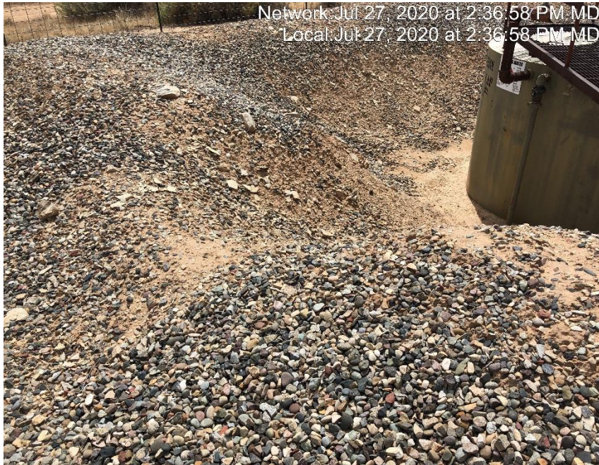
Photo #1627 Secondary containment berm has eroded.
