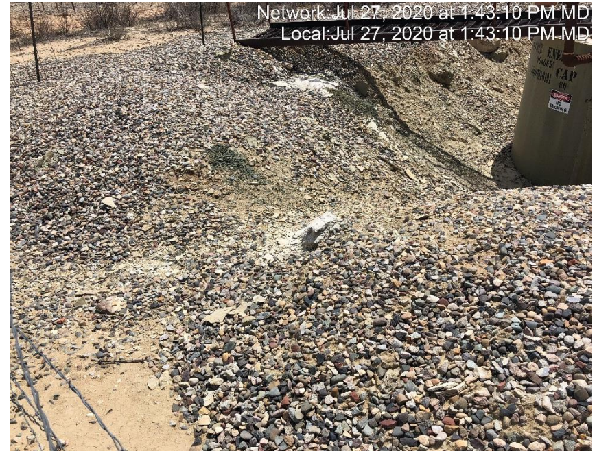
Photo #1624 Secondary containment berm has eroded.
