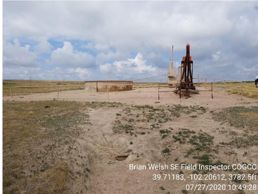
1. Wellhead and erosion leading to the east off of location
