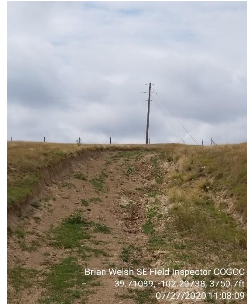
2. Erosion on access
