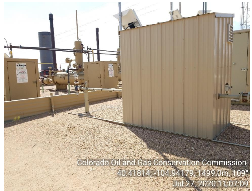
Photo 8: Disconnected/unused gas meter
