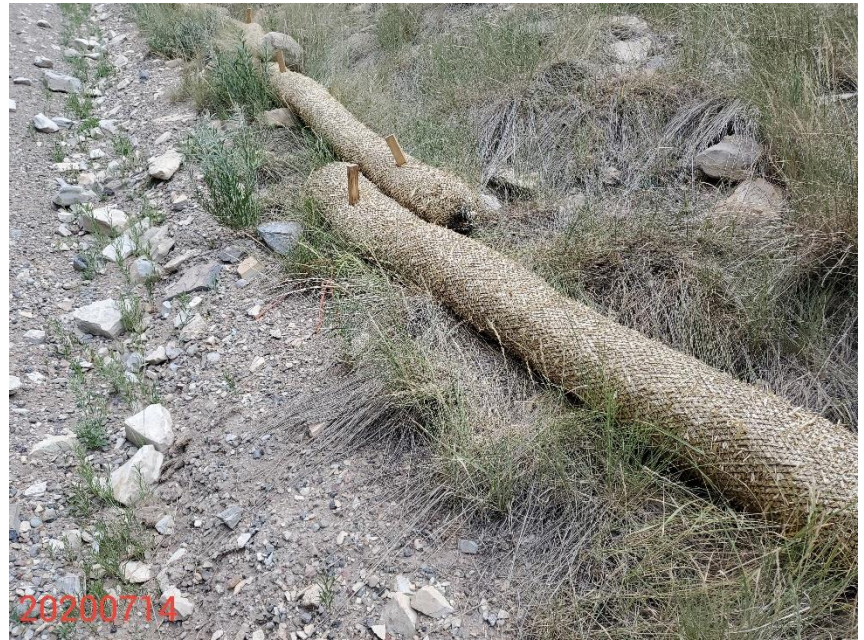
Photo 12: Photo taken from the access road, west of the Location facing north. Photo shows Operator implemented straw wattles along perimeter of the Location. Photo shows BMP has not been installed in accordance with good engineering practices and is not in proper functioning condition; Wattles require trenching and backfilling.
