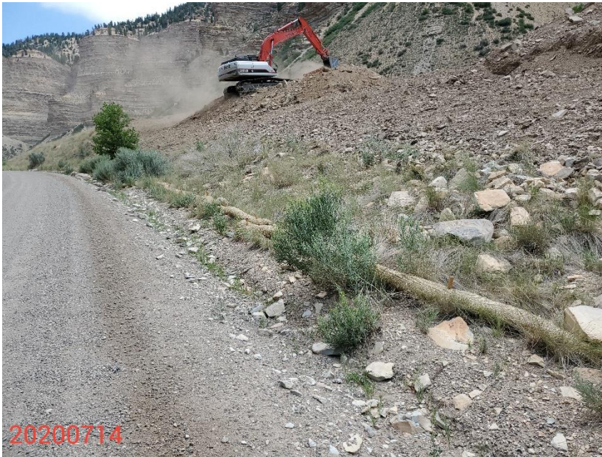
Photo 11: Photo taken from the access road, west of the Location facing north. Photo shows Operator implemented straw wattles along perimeter of the Location. Photo shows BMP has not been installed in accordance with good engineering practices and is not in proper functioning condition.
