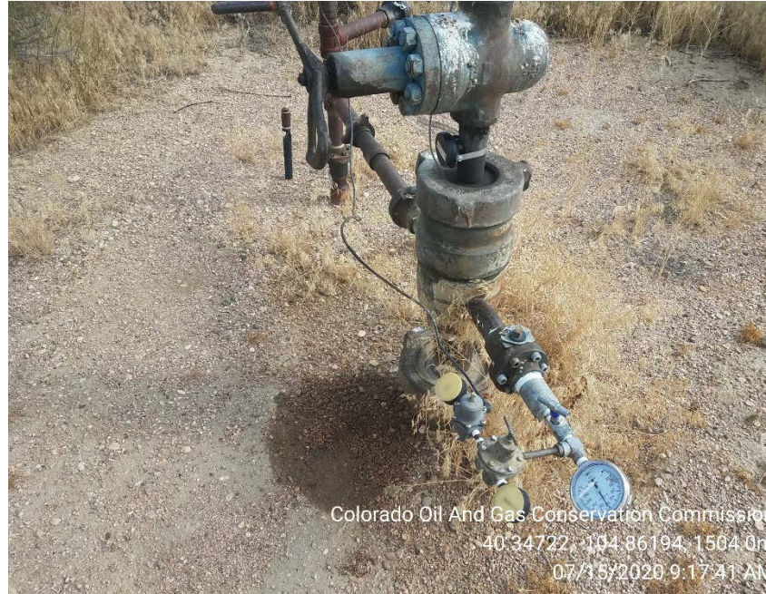
Master valve leak and stained soil
