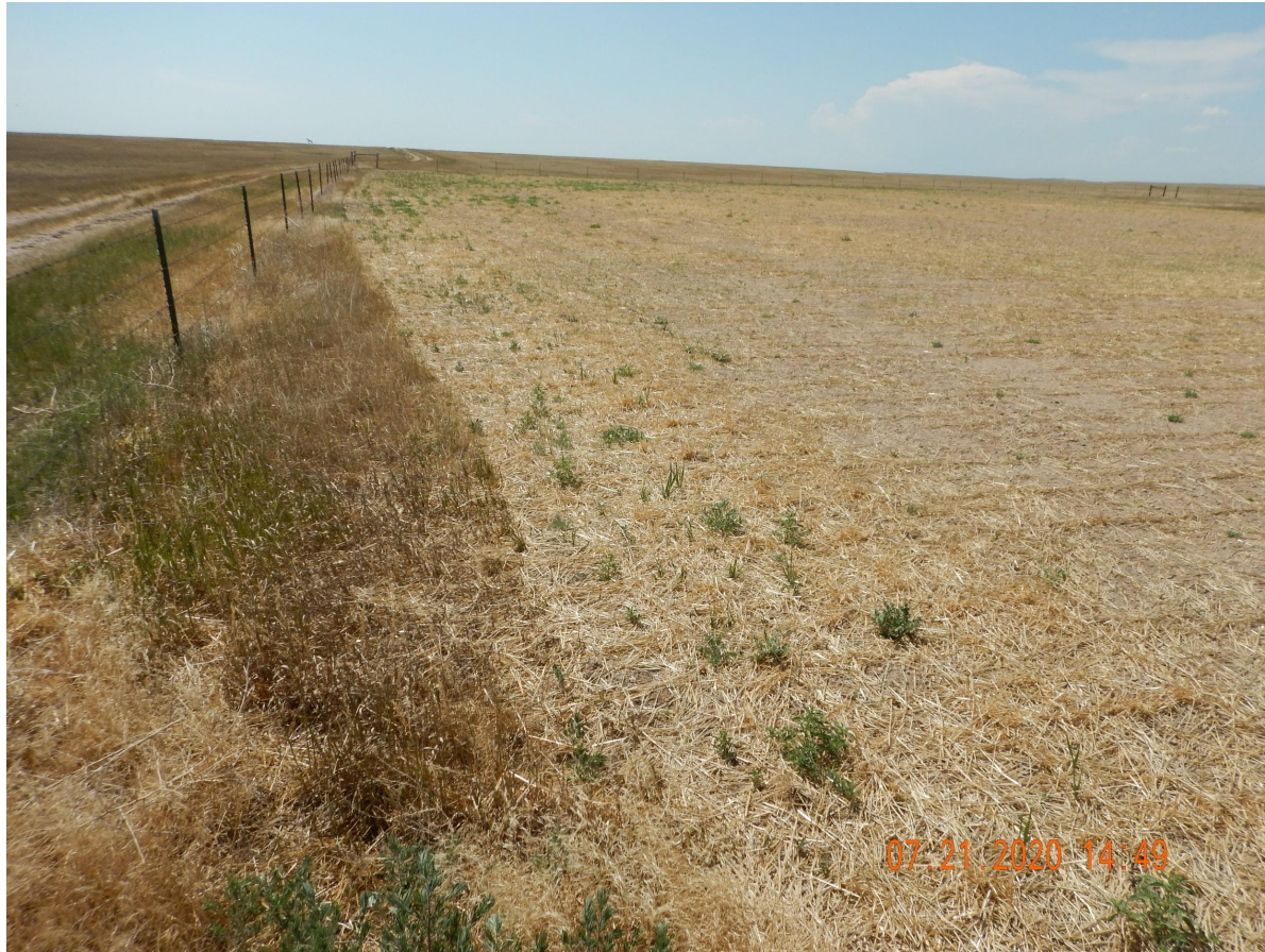
Photo 1. Photo taken from the entrance to location, facing West. Photo illustrates the Operator has performed final reclamation activities with the evidence of straw crimped mulch and drill rows.
